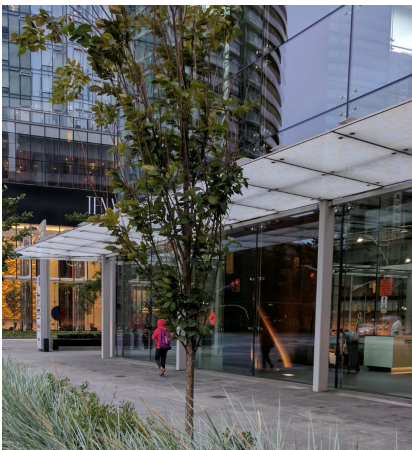
Figure 29: One York St. Cantilever Treatment
