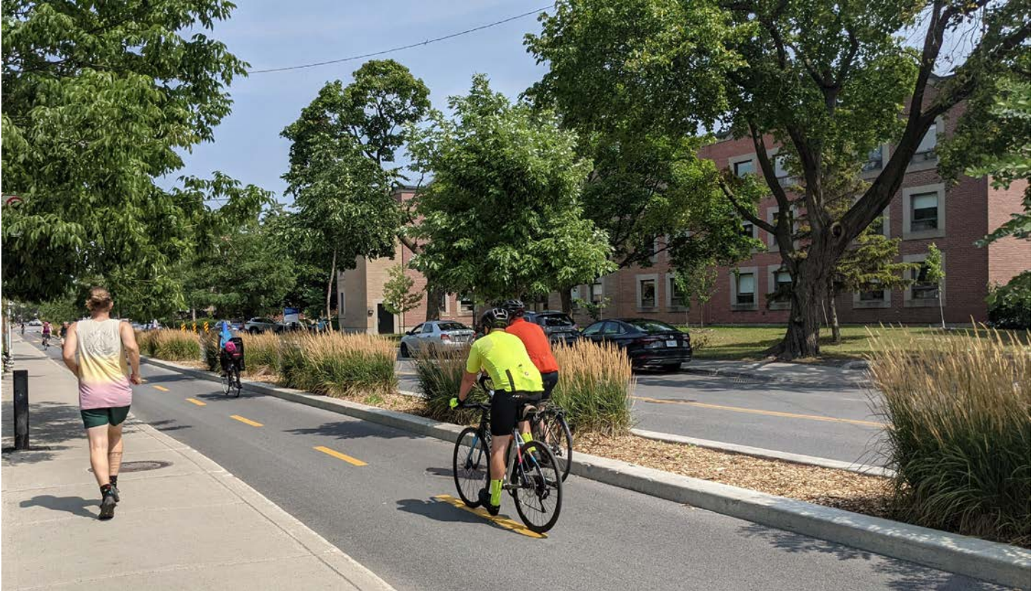
Two-way cycle tracks protected by wide landscaped buffers provide enhanced safety and comfort for cyclists of all ages and abilities (Brook McIlroy).
