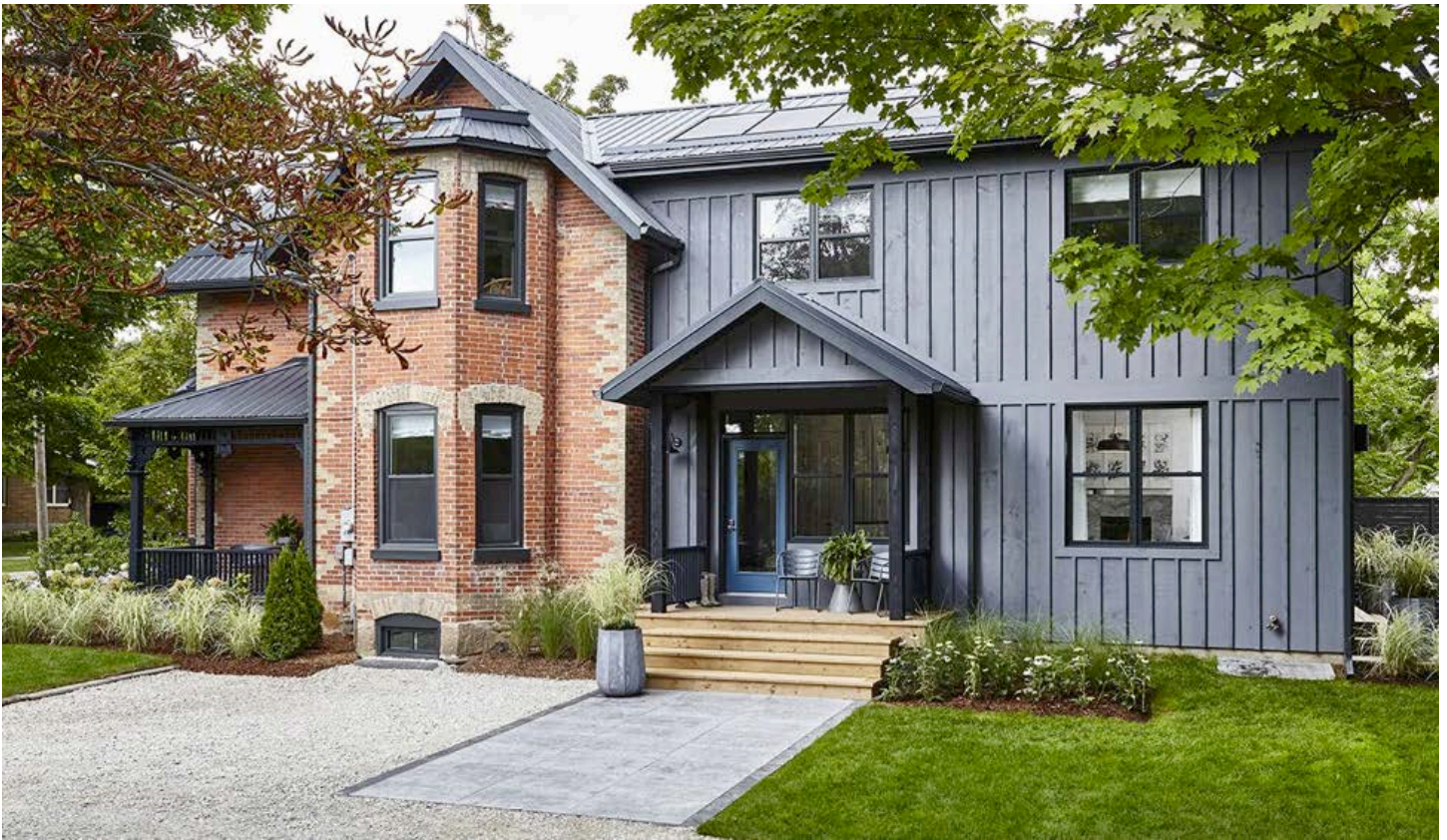
Additions to built heritage resources should respond to the heights and proportions of the existing building (Sarah Richardson).
