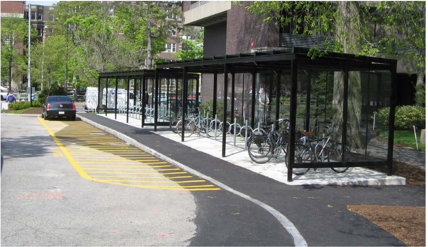
Sheltered bicycle parking area (Lucid Management).
