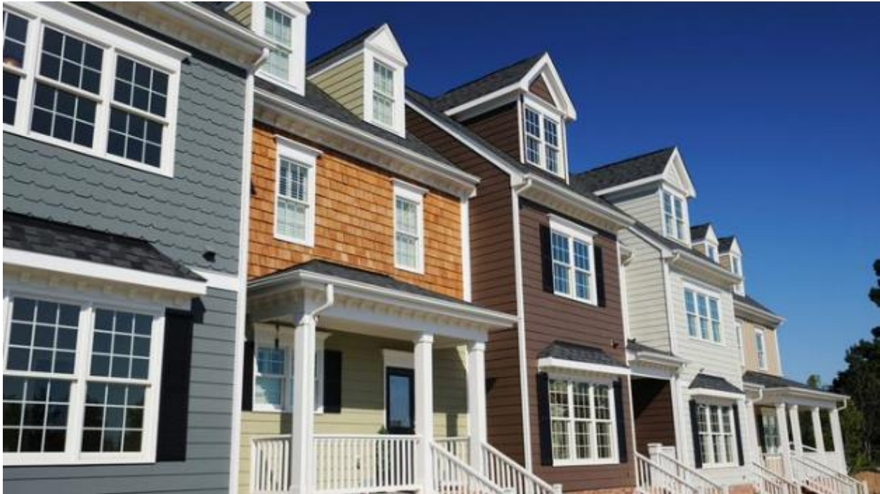
Figure 33. Articulation can break up the massing of housing blocks and provide visual interest (Realtor.com).
