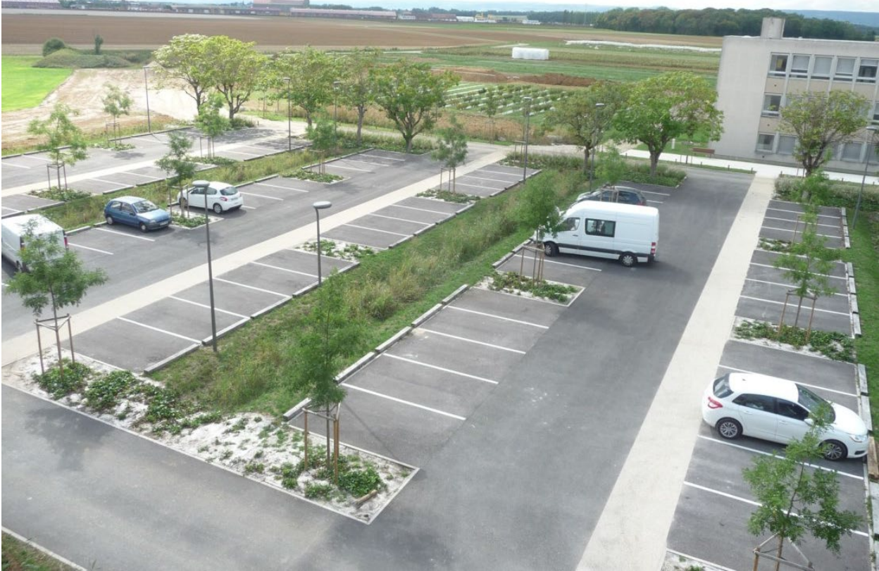
Figure 38. The surface parking lot above includes bioswales and tree plantings to improve stormwater management (Mayot & Toussaint Paysagistes).
