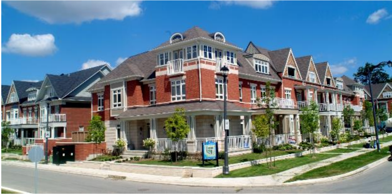
Figure 32. Buildings on corner sites should address each street edge with comparable architectural design (Brook McIlroy).
