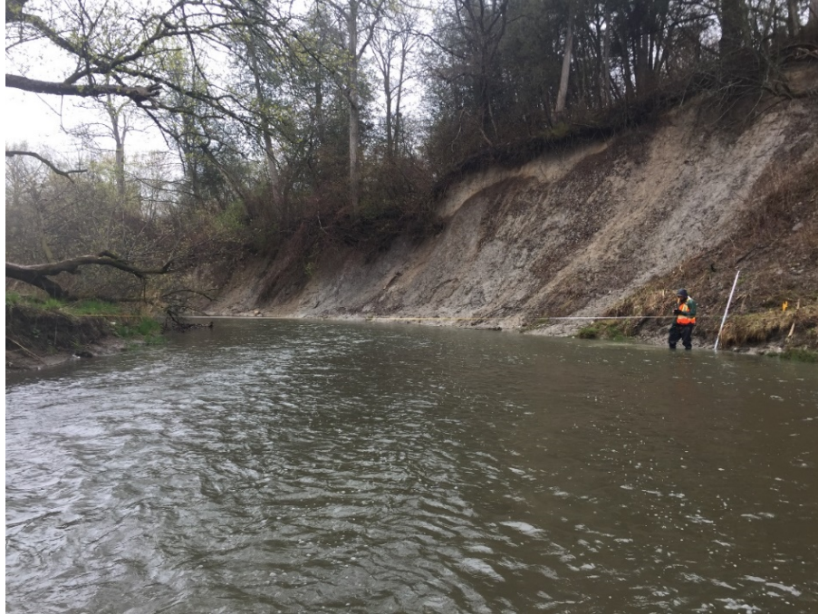
Photo 9. An actively eroding scarp, approximately 100 m long and up to 17 m high, along the western valley wall at Site 6. Downstream view.
