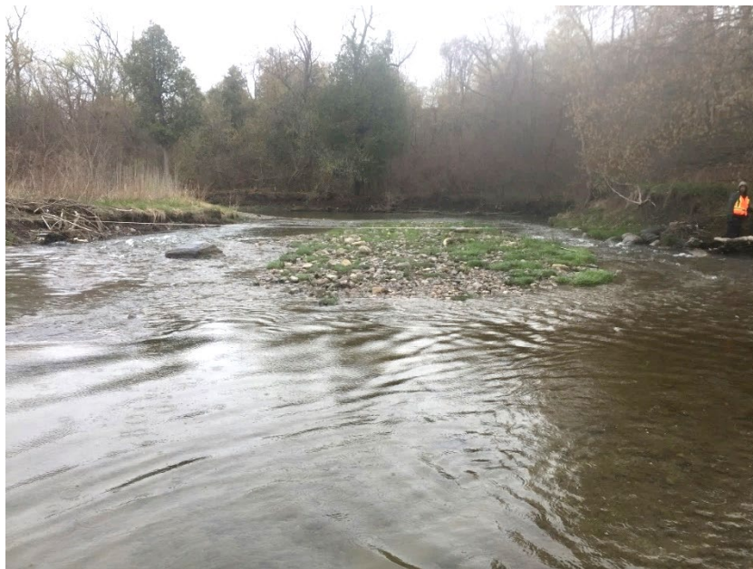
Photo 8. A medial bar overtop of the sanitary sewer bifurcates flow, concentrating erosion along both banks. Downstream view.
