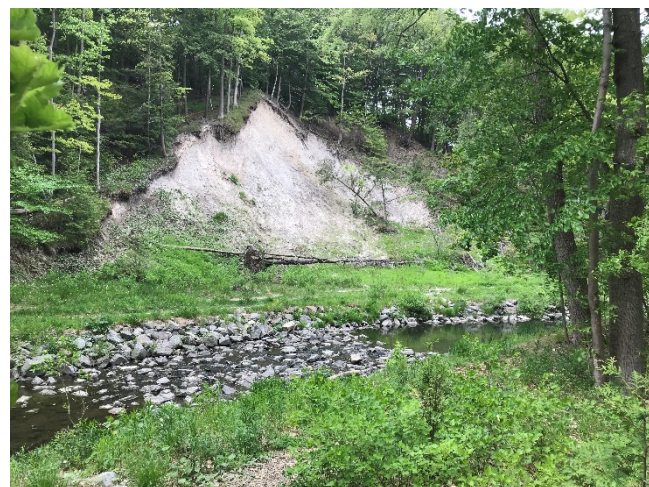
Photo 12. Example of boulder-protected, slope-toe bench constructed along Wilket Creek, Toronto.
