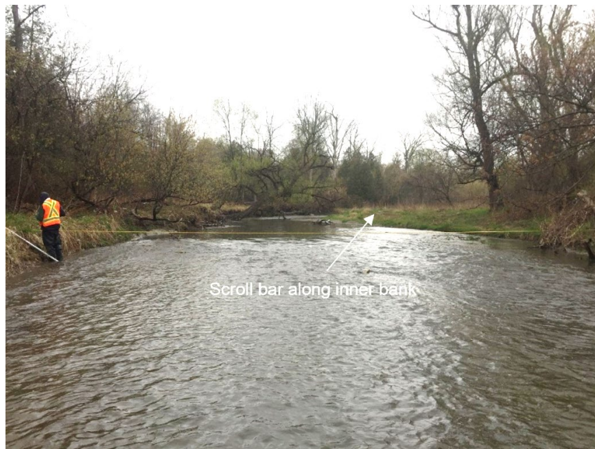
Photo 11. Upstream view of channel approaching Site 6. A low, gentle eastern bank maintains good floodplain connectivity and helps attenuate flood energy. Upstream view.
