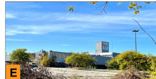
Former Knob Hill Terminal, Oshawa
