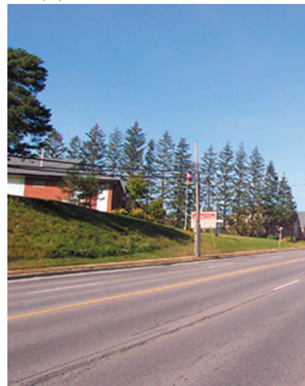
Looking north along the study corridor with the Shrine Club on the west side
