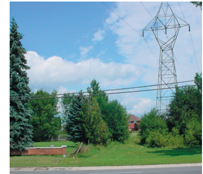
About 100 metres south of Conlin Rd. E. is a hydro corridor which crosses Simcoe St. N. along an easement over public and private lands
