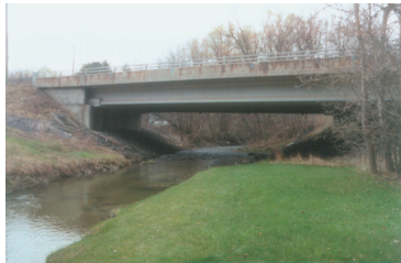
Downstream (west) view of bridge over Oshawa Creek
