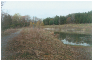
Stormwater management pond on northwest overbank
