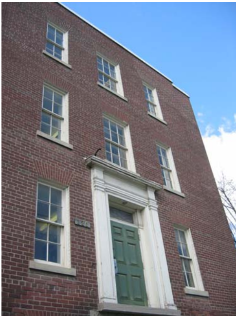
2. McLaughlin Hall, Original Entrance, East façade, April 2006
