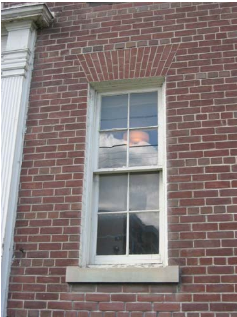
4. McLaughlin Hall, Window Sash – East façade, April 2006
