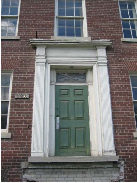
5. McLaughlin Hall Entrance, South façade, April 2006
