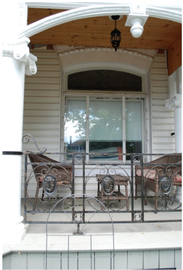
4. Metal Railing Detail and Archway
