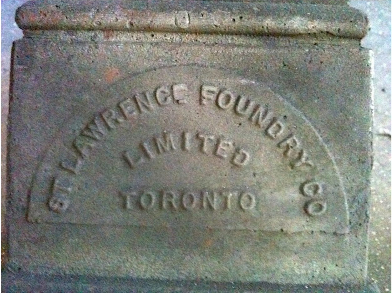
2. Foundry Stone originally located on each end of the verandah railing as a support.
