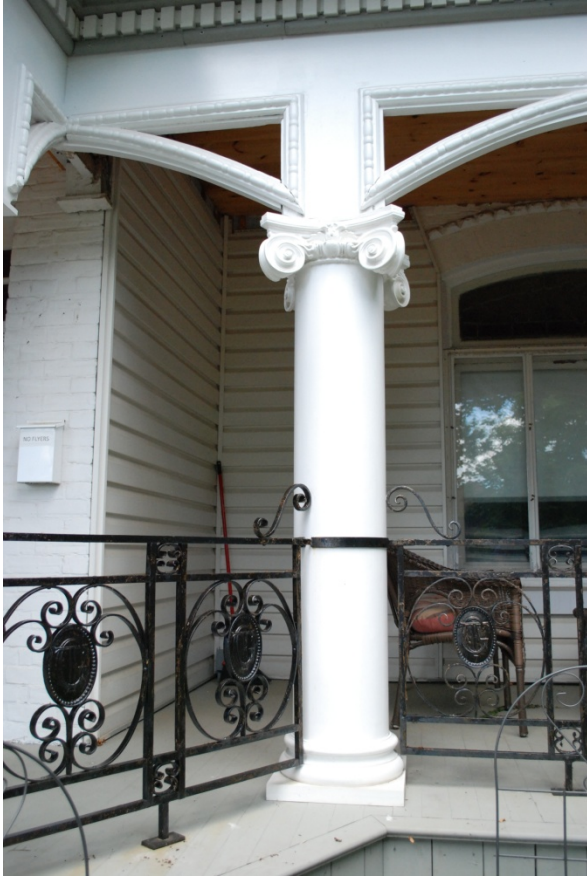
3. Verandah Detail, south façade
