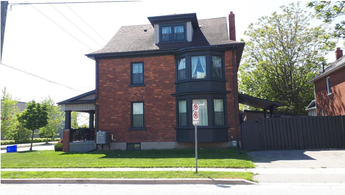
Figure 9 - 122 Division, north façade, May 2021
