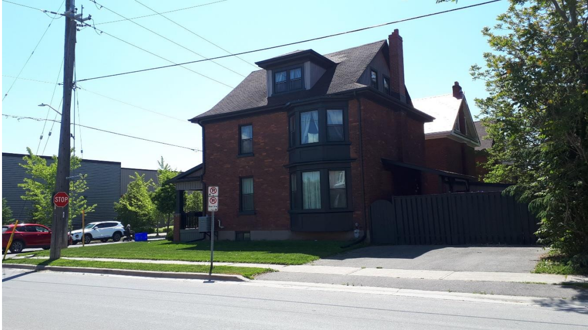
Figure 10 - 122 Division Street, northwest façade, May 2021
