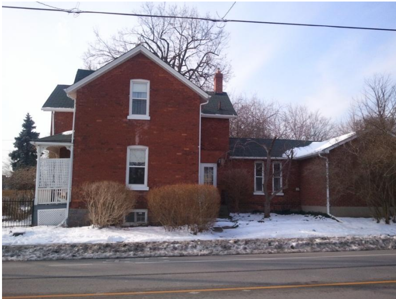
East Façade showing additions on the north facade, 76 Elgin Street East, January 2013
