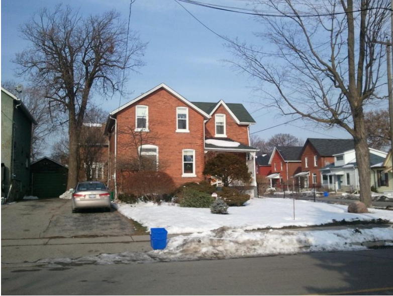
Main Façade, South Façade, 76 Elgin Street East, January 2013
