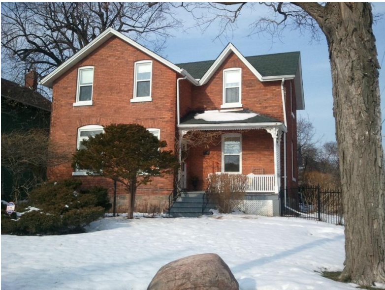
South Façade, 76 Elgin Street East, January 2013
