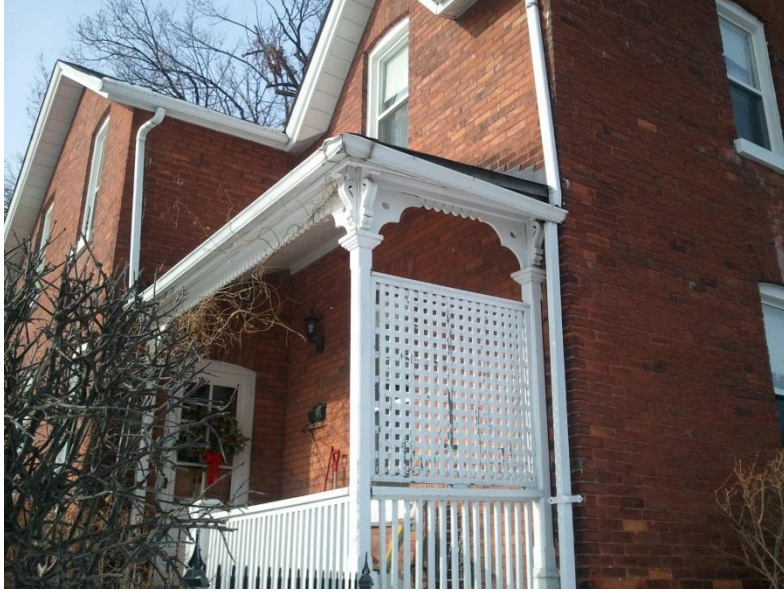
Porch, South Façade, 76 Elgin Street East, January 2013
