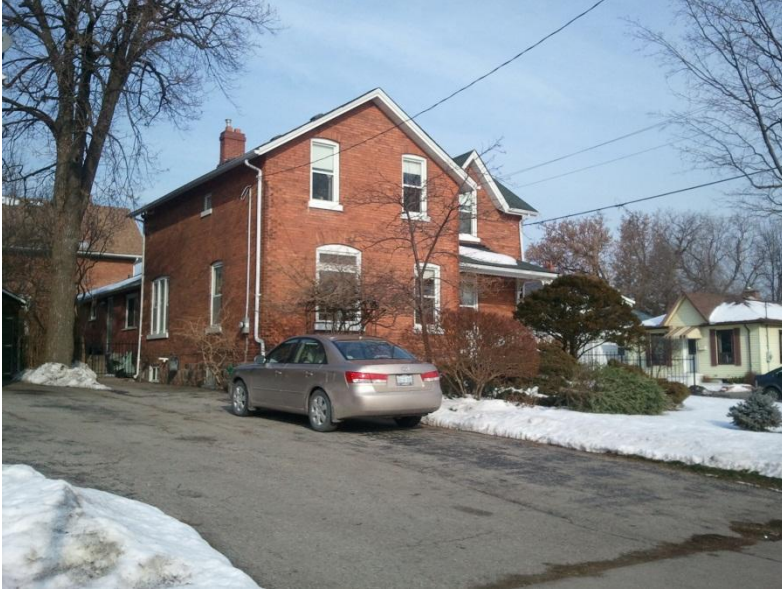
Southwest Façade, 76 Elgin Street East, January 2013
