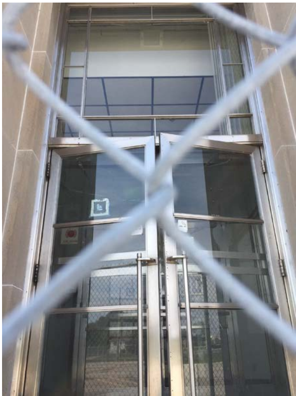
Figure 8 - 700 Park Road South, close-up view of of main entrance with stainless doors and transom (left); and (right) window to left of door with stainless framing and lower panel.
