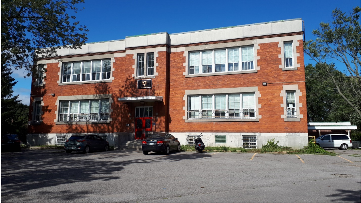
Figure 8 – 827 Gordon Street, Oshawa, ON, west façade, August 2021
