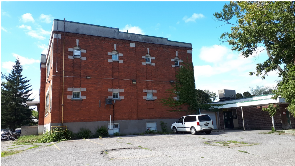
Figure 9 – 827 Gordon Street, Oshawa, ON, south façade, August 2021
