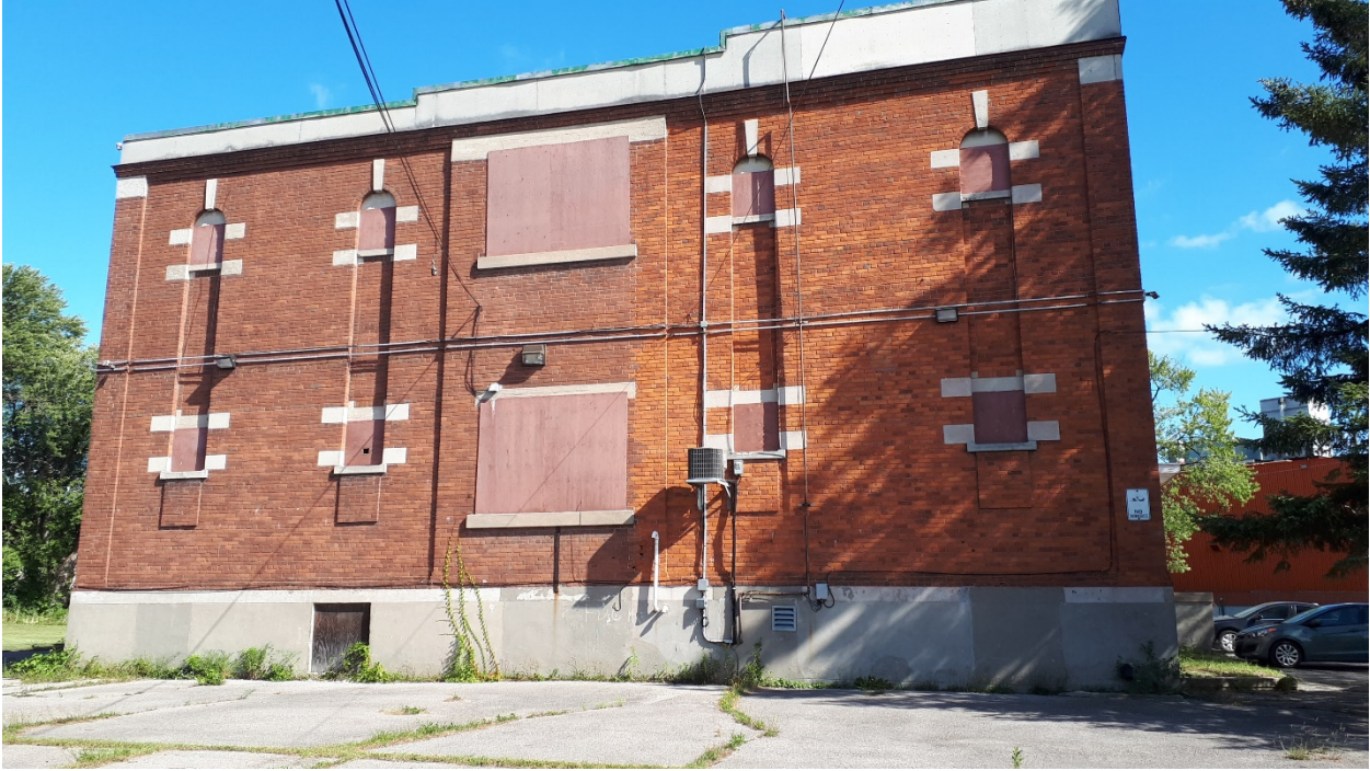
Figure 10 – 827 Gordon Street, Oshawa, ON. north façade, August 2021
