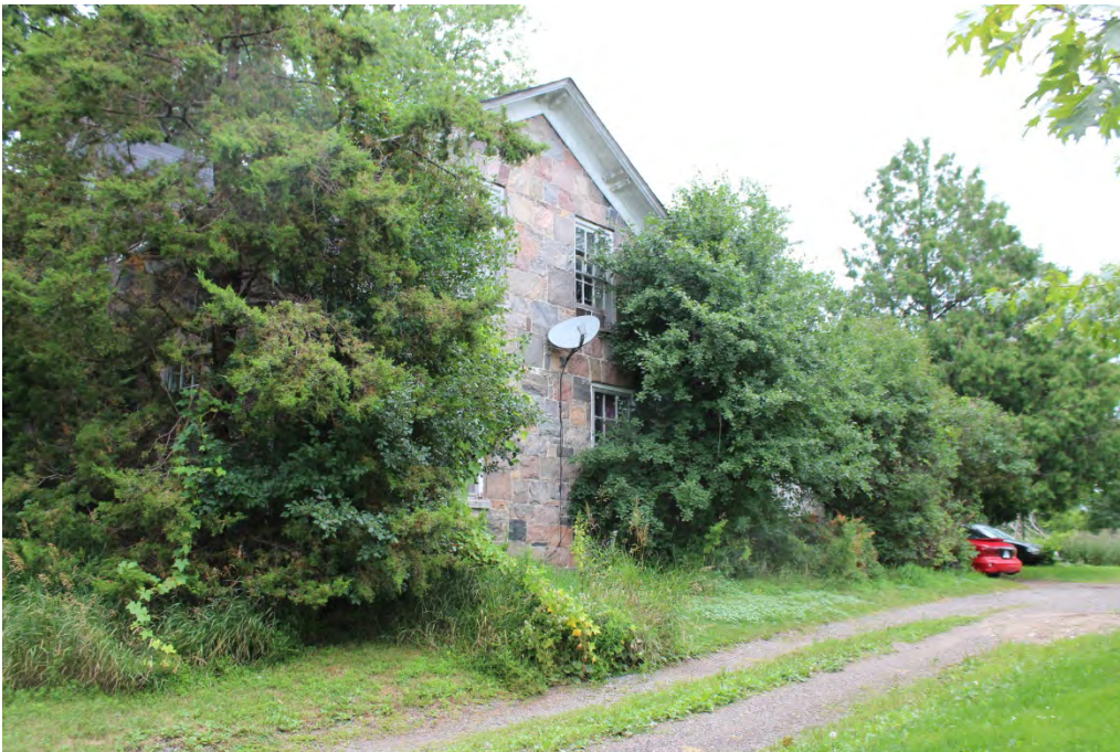
2. 2651 Harmony Road North, South Elevation
