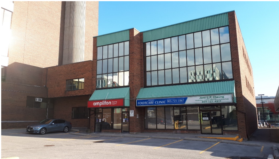
Figure 14 – 117 King Street East, three-storey west wing addition, north façade, May 2021
