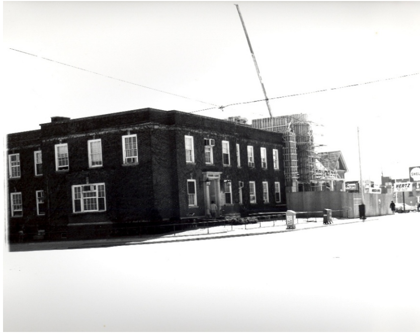
Figure 7- Facing South-West, this photograph shows the construction of the tower addition to the Oshawa Clinic. The original clinic building is the two storey one at the left of the photograph. Image: Thomas Bouckley Collection, RMG. 1970
