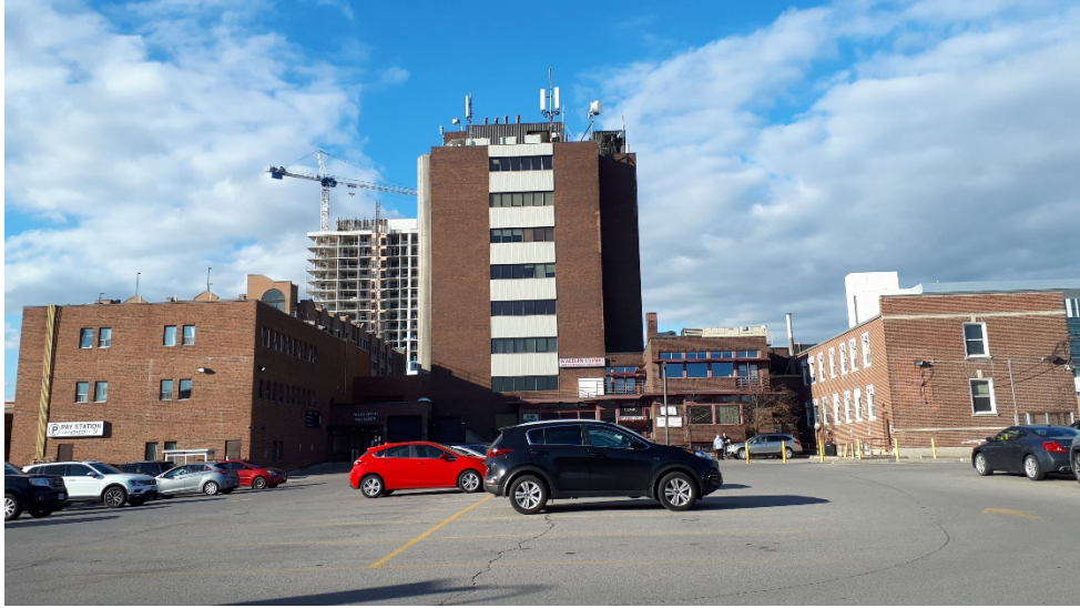
Figure 15 - 117 King Street East, east façade and parking lot, May 2021
