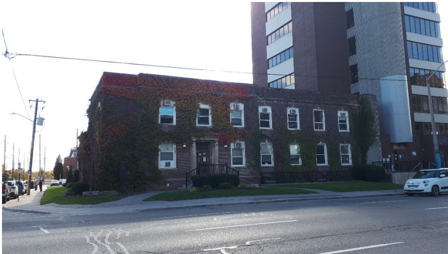
Figure 12 – 117 King Street East, north façade, original Clinic Building constructed in 1948. October 2021
