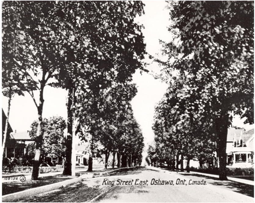
Figure 6 - Houses on the left side of the photo (the north side of King Street east) include F.L.Fowke's residence, W.E.Eaton home, hidden by a tree, Dr.Henry's residence, and the R.S.McLaughlin home. Houses at the right were demolished to make way for the Oshawa Clinic. Image: Thomas Bouckley Collection, RMG. Circa 1905.
