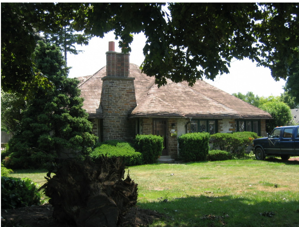
2. 469 King Street East, North Façade – June 2007
