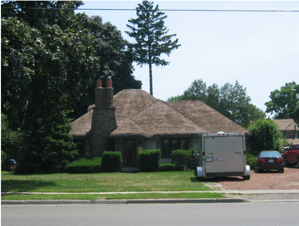
1. 469 King Street East, North Façade – June 2007
