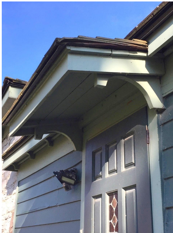
The porch shed roof on the west elevation "tail" of the house, showing the simple but elegant supporting brackets.
