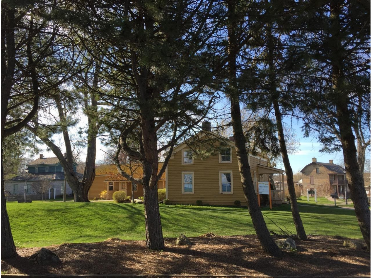
View of Henry House (left), Guy House (centre), and Robinson House (right) looking north from Lakeview Park.
