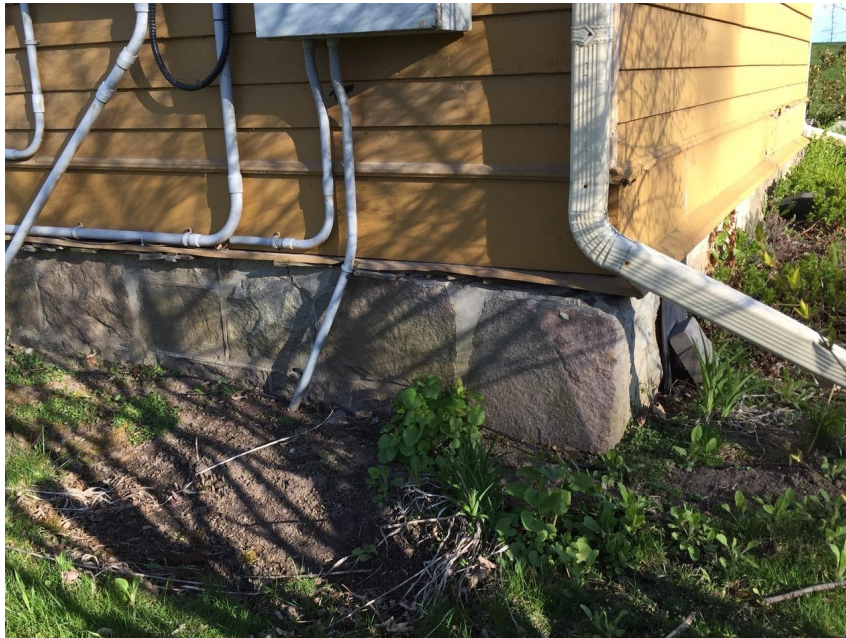
Guy House foundations, likely fieldstone
