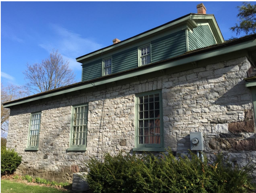
View of north elevation with limestone walls and 12-over-12 first-storey windows.
