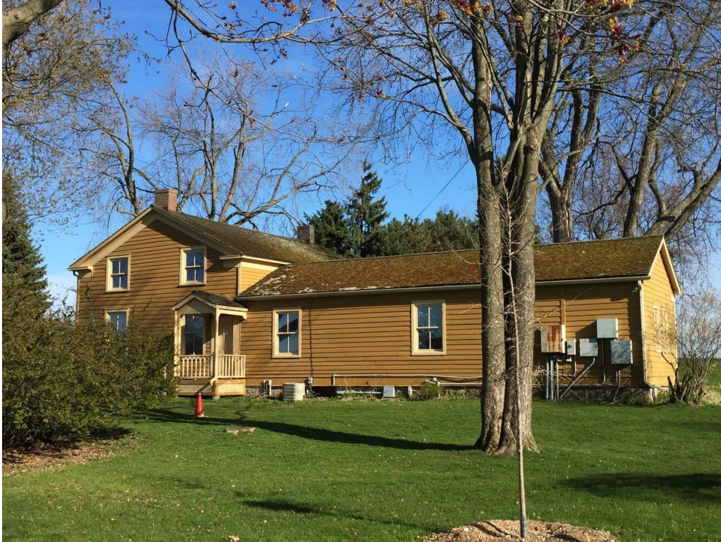
Guy House, north elevation
