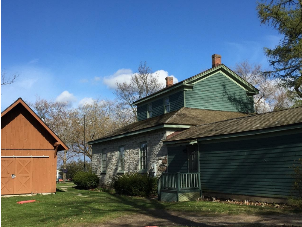
North and west elevations, Henry House and drive shed
