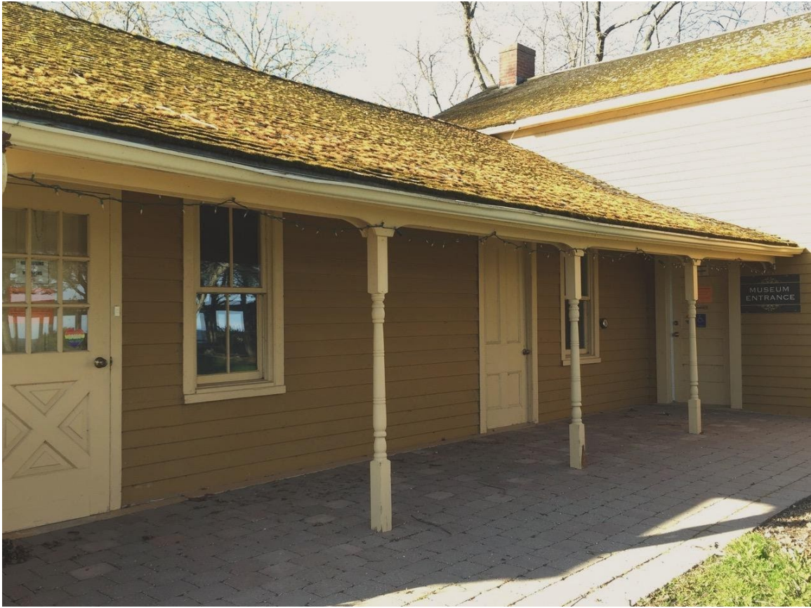
Guy House south elevation with galleried porch and turned posts
