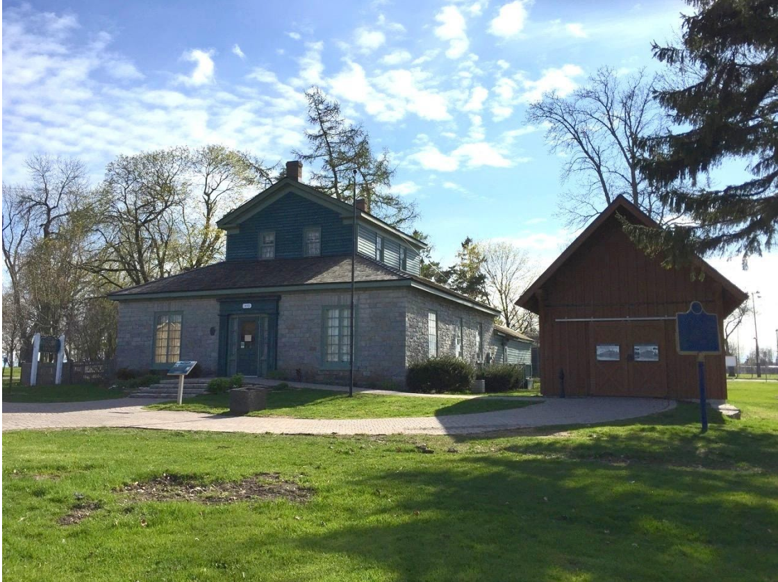
Henry House east façade and Drive Shed
