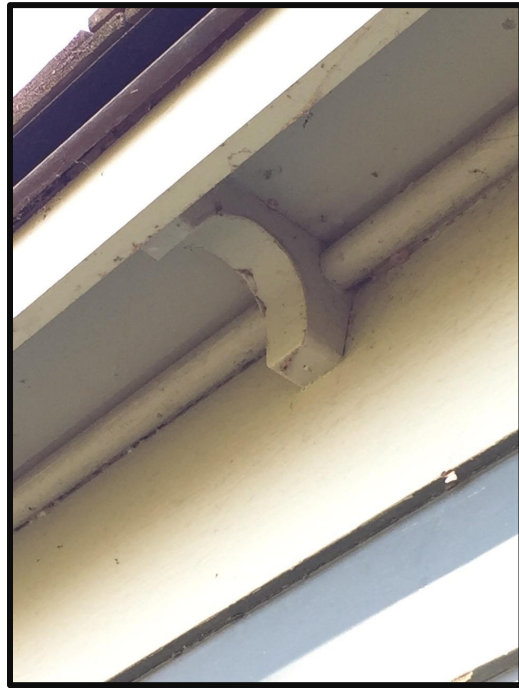
The simpler but still decorative cornice brackets used on the "tail" of the house.
