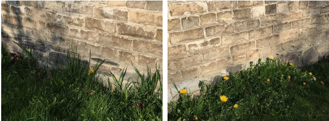
Robinson House foundations, likely fieldstone
