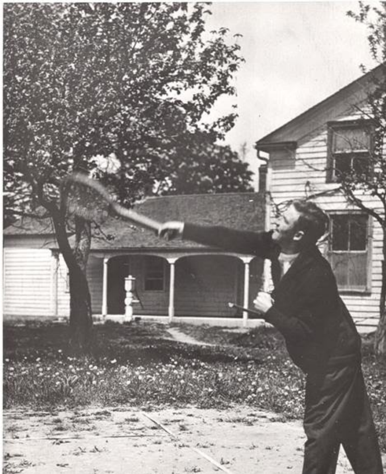
The Oshawa-on-the-Lake tennis court was directly south of Guy House. This 1930 photo shows many of the house's features have survived. Note the well hand-pump. R.M.G. Thomas Bouckley Collection.
