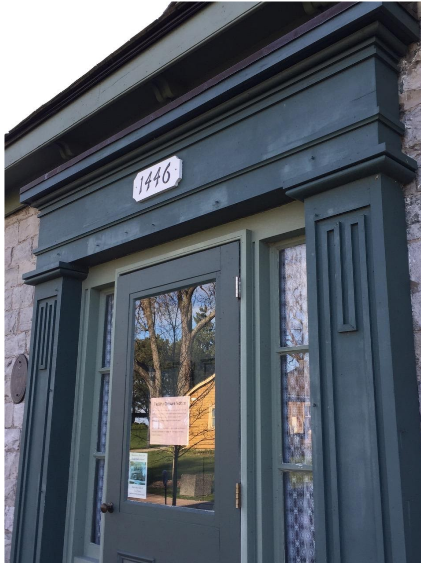
Henry House front entrance with side lights, decorative pilasters, and entablature
