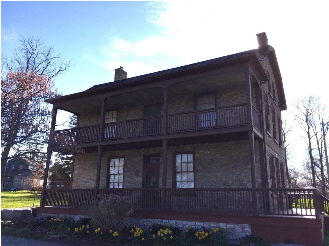
Robinson House, south elevation
