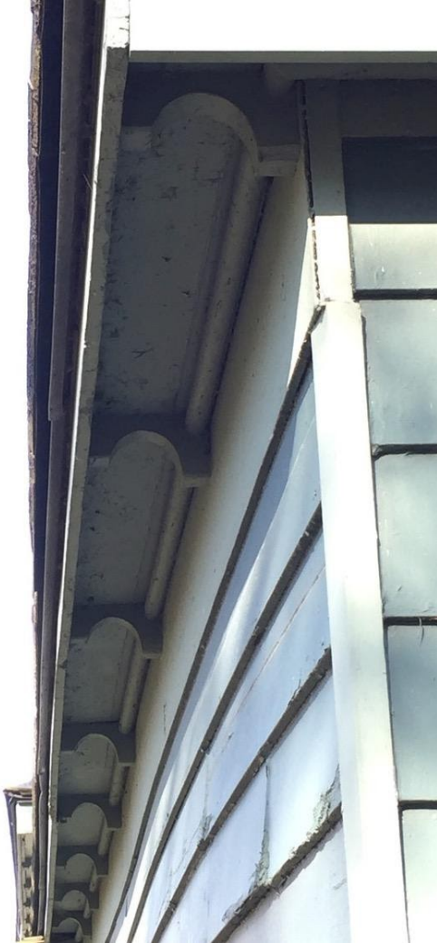
The simpler but still decorative cornice brackets used on the "tail" of the house.
