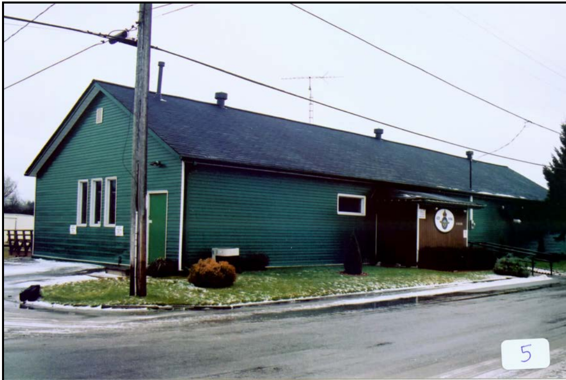
Photograph No 5 North and west facades
