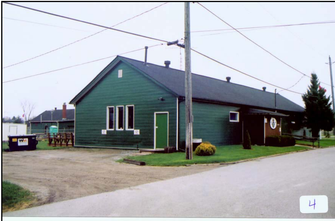
Photograph No 4 North and west facades
