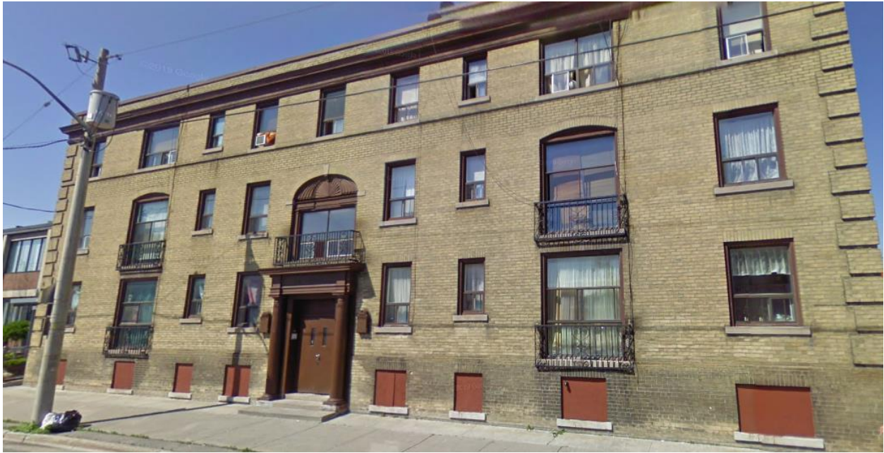
Figure 11 - 304 Simcoe Street South, The George, pre-restoration (June 2009), Google Street View Image
