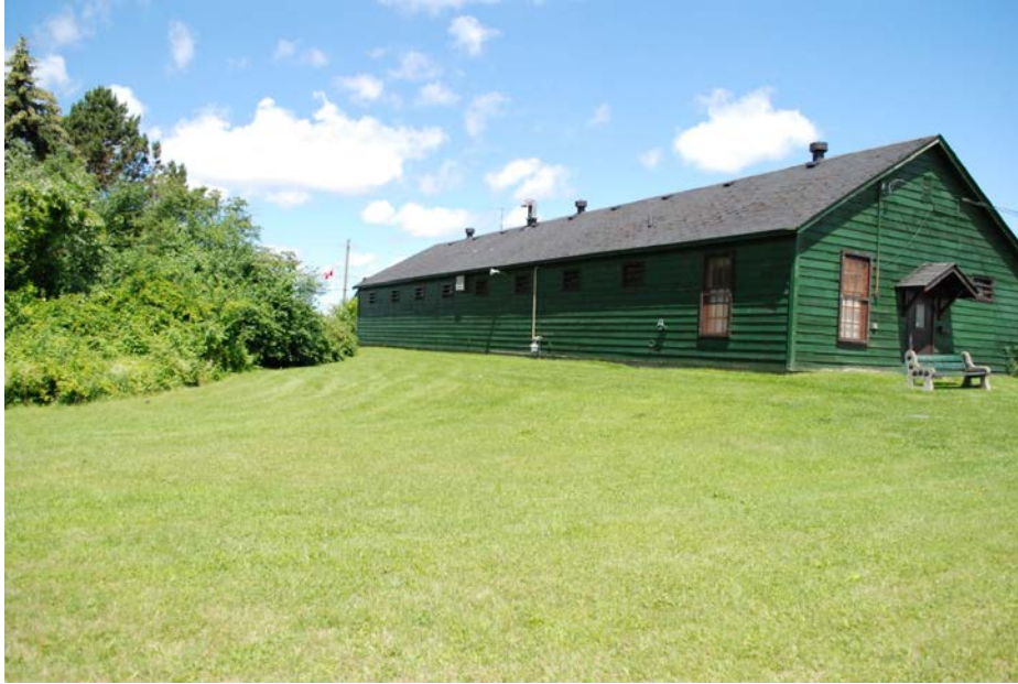
7. South Facade, Former Stores Building
