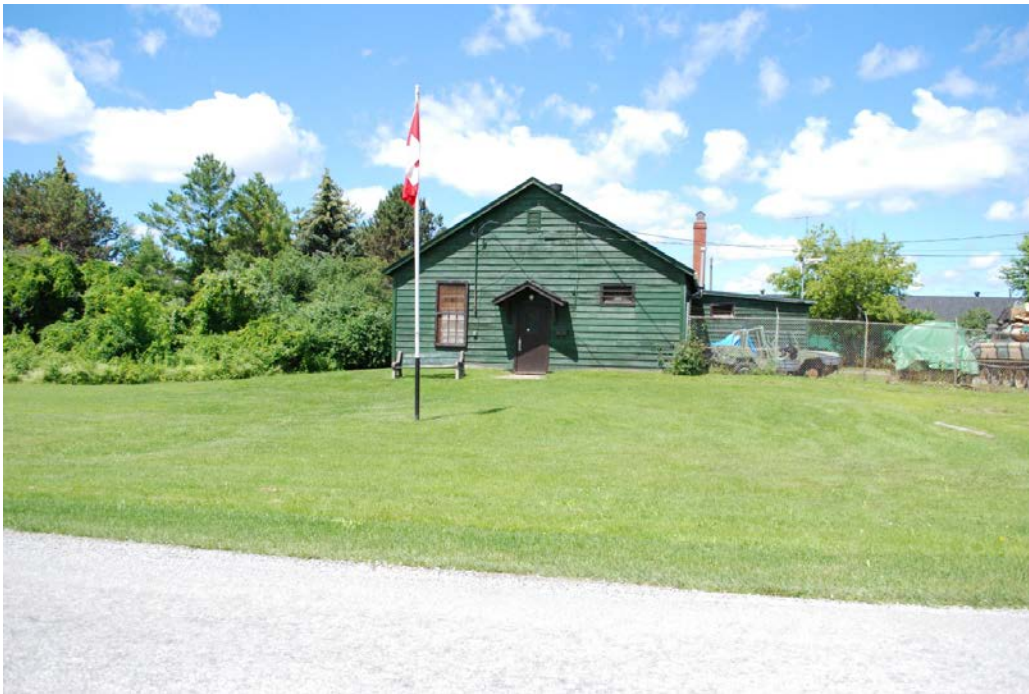
6. East Facade, Former Stores Building
