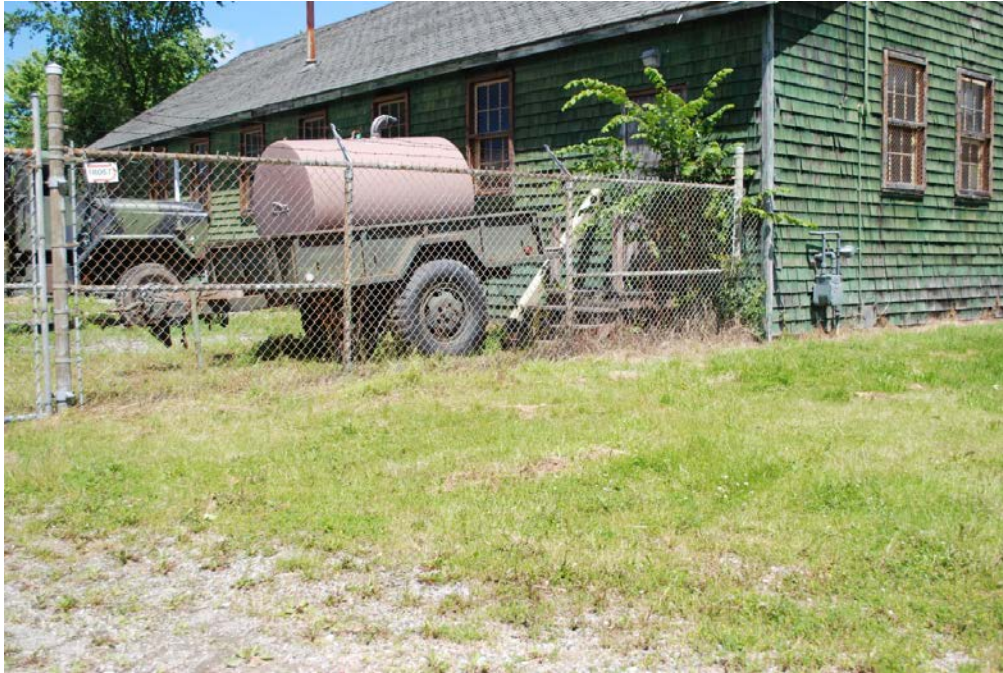
3. South Facade, Former Canteen. Entranceway and 6 windows featuring 6 over 6 paned windows.
