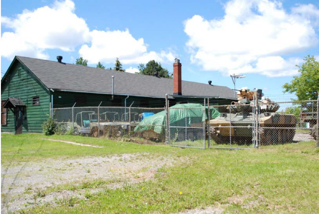
9. North Facade and Vehicle Compound, Former Stores Building
