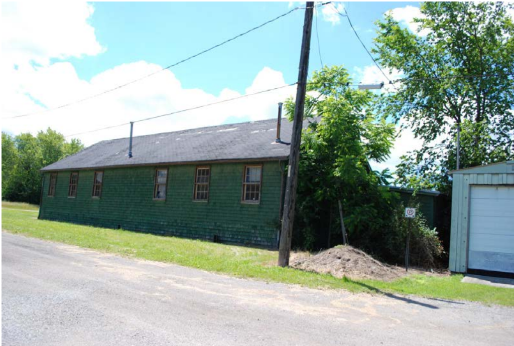
4. North and West Facade, Former Canteen.
