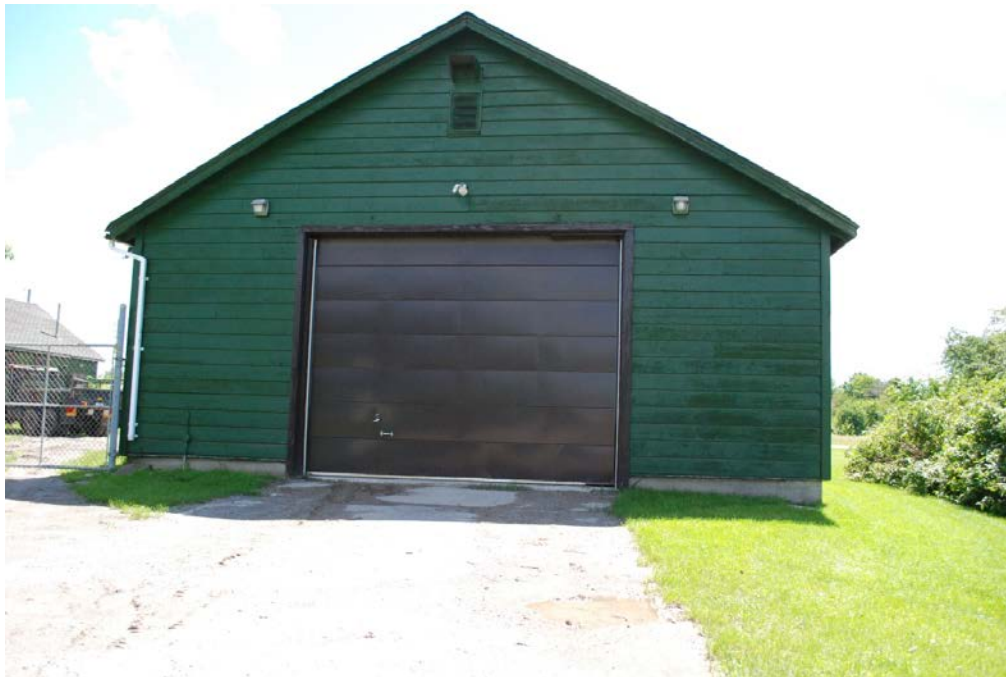
8. West Facade, Former Stores Building
