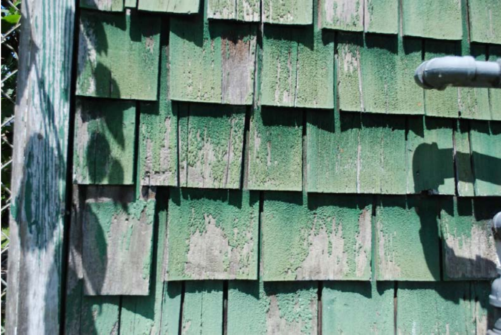
5. Close up of original cedar shingle cladding on the former Canteen building.
