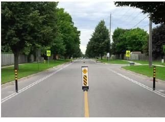
Example of a flexible bollard with delineators
