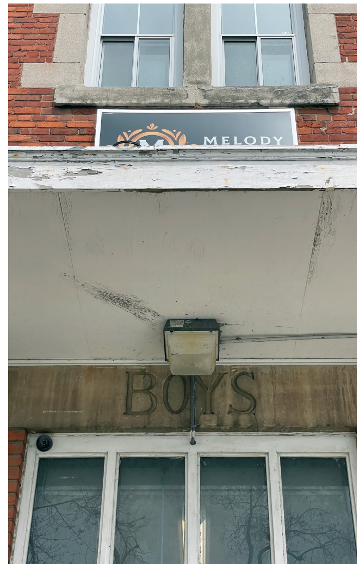
Figure 7: Original boys entrance at the southwest facade. EVOQ.
