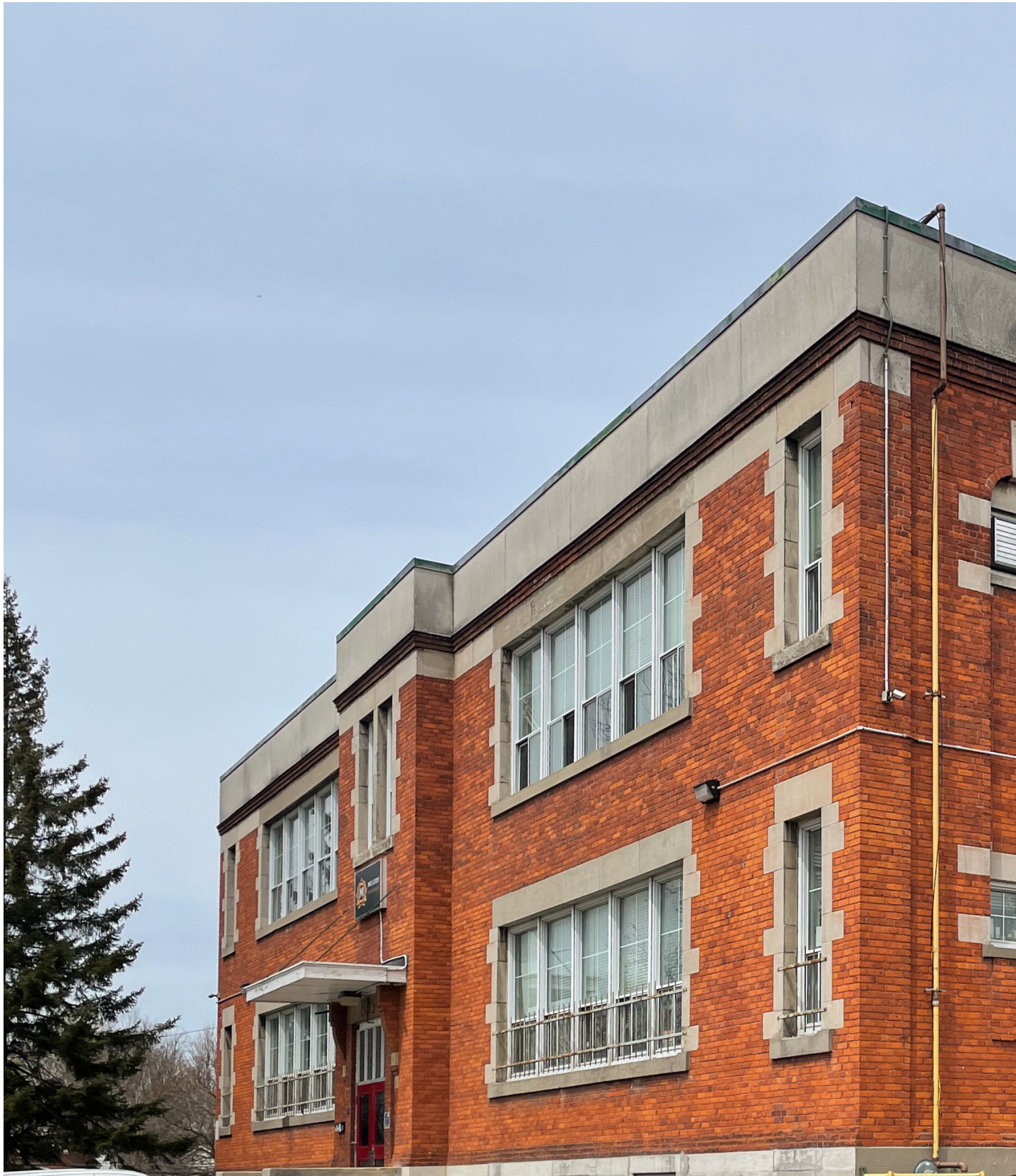
Figure 1: View of southwest (main) elevation. EVOQ.
