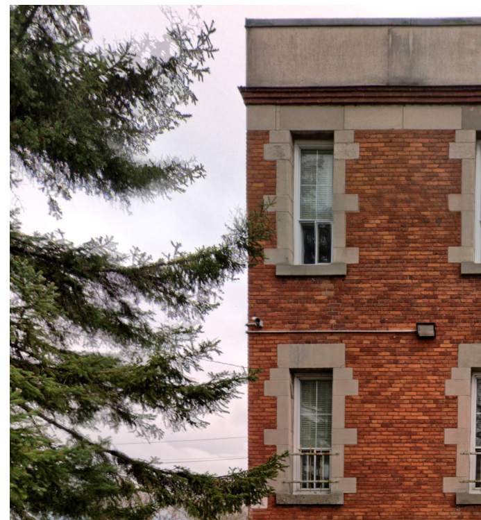
Figure 24: Window details, southwest facade. EVOQ.
