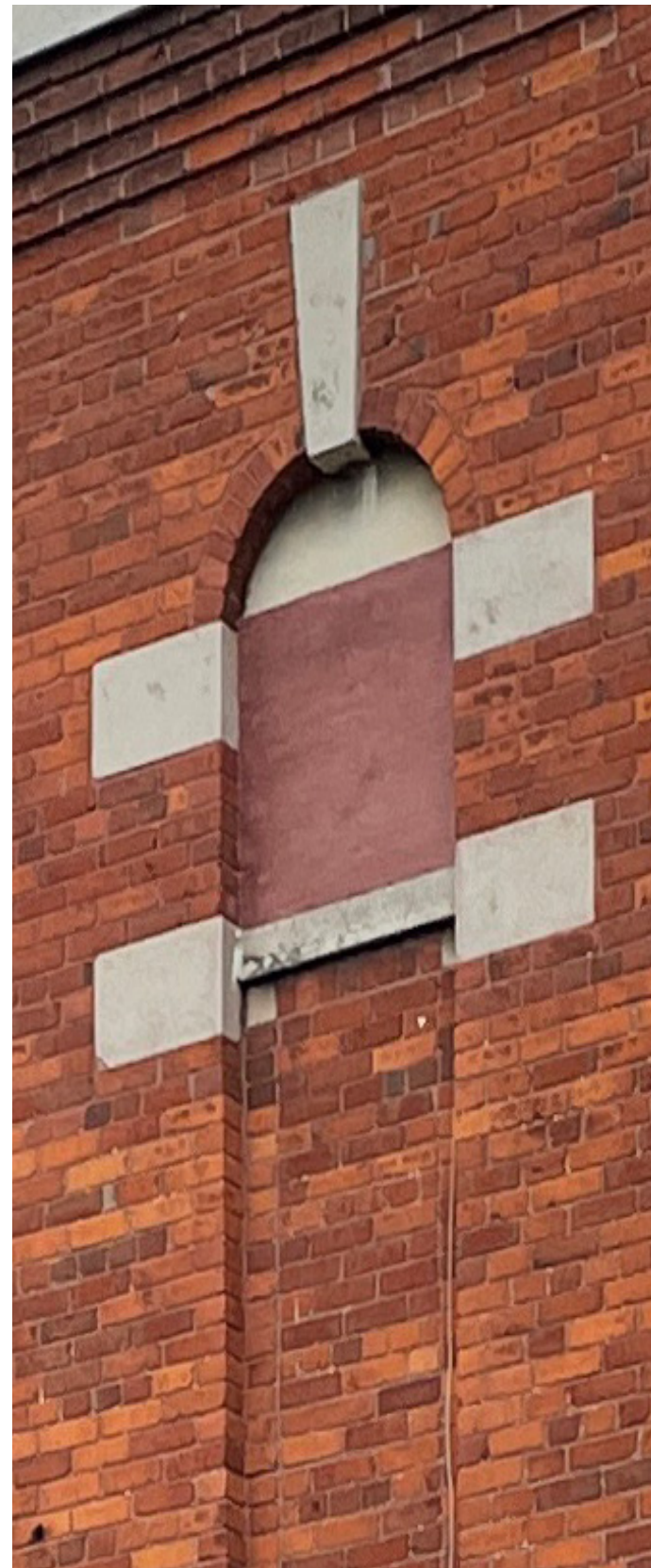
Figure 4: Brick and stone detailing around recessed window (boarded). EVOQ.
