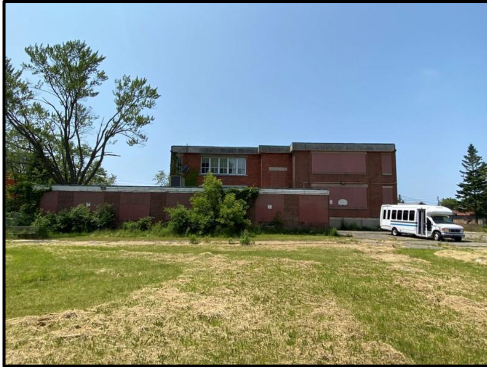
Image 5: North Elevation and Rear Addition and 827 Gordon Street (Photo taken on June 19, 2023; Facing South)
