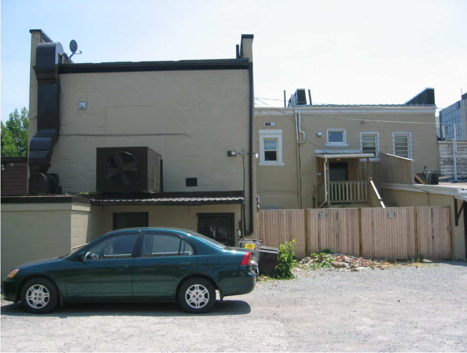
1. 10-14 Bond Street West, North Façade – June 2007
