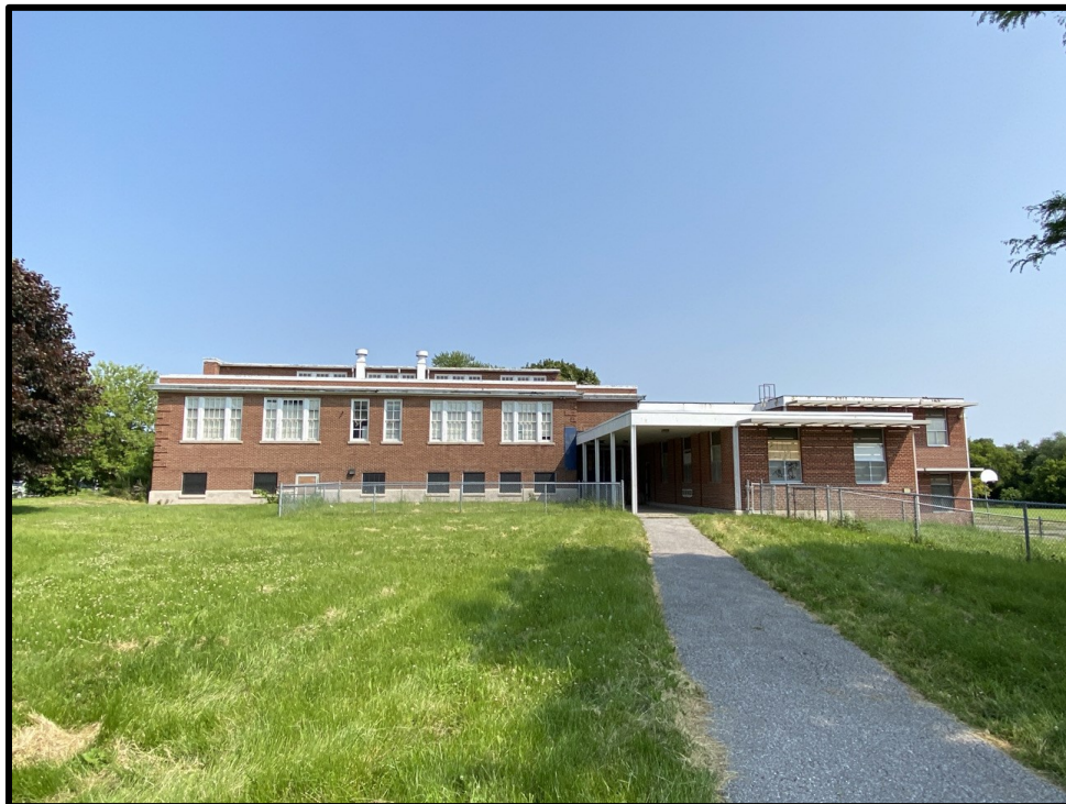
Image 4: South Elevation of 149 Harmony Road South (Photo taken June 19, 2023; Facing North)
