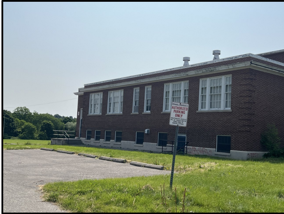
Image 5: North Elevation of 149 Harmony Road South (Photo taken on June 19, 2023; Facing Southeast)
