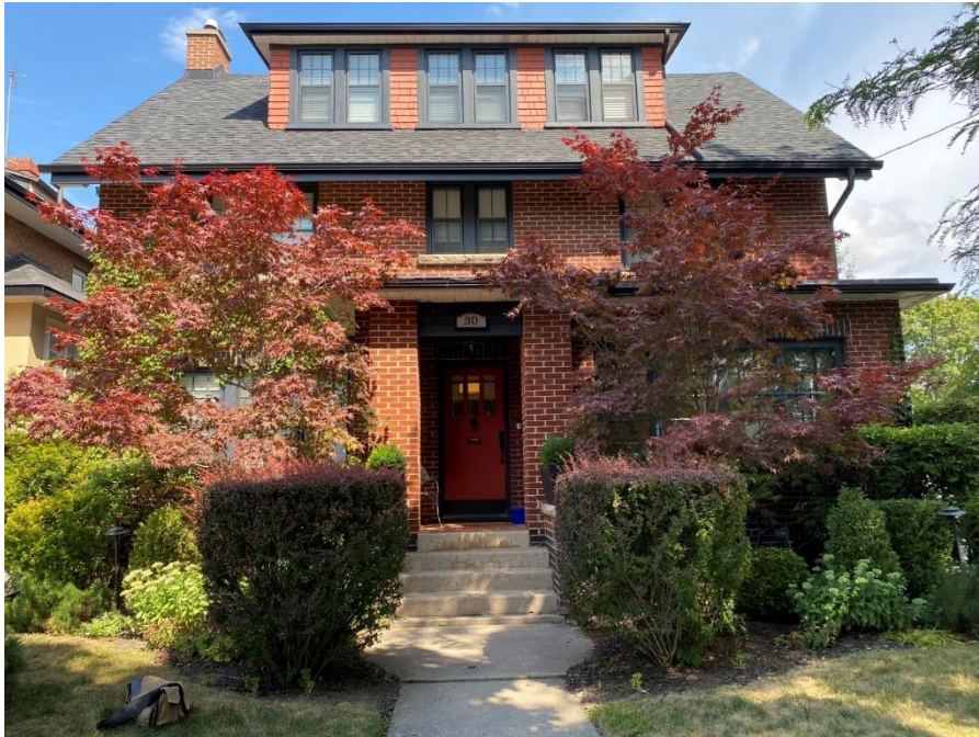
Figure 22: Front façade (southern elevation) (A.S.I. 2022).
