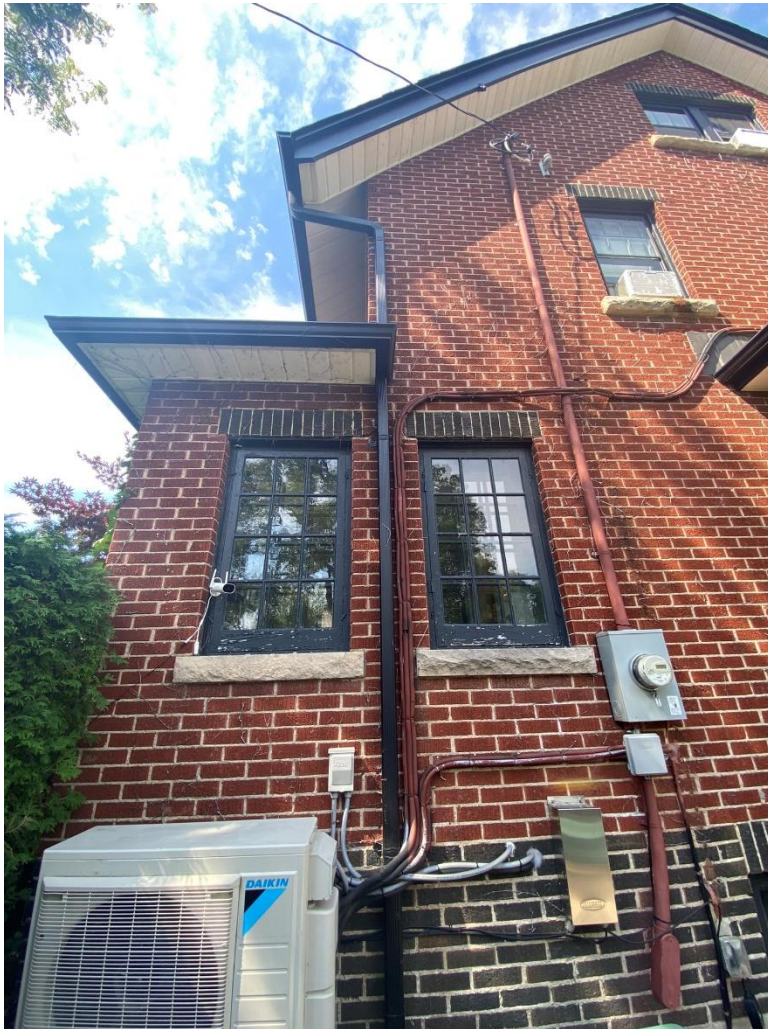
Figure 28: View of the decorative brickwork and concrete lug sills along the windows along the eastern elevation (A.S.I. 2022).
