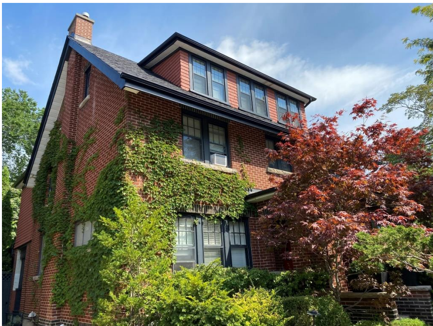
Figure 27: Detail view of the repeating fenestration pattern along the front façade (A.S.I. 2022).
