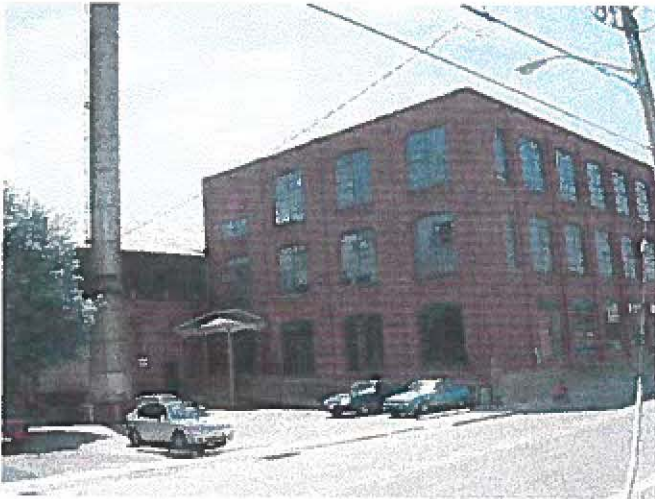
6. Alger Press, East façade of Building, May 2006
