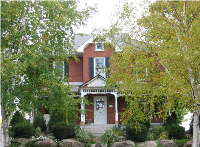
1. Pascoe House, West Façade
