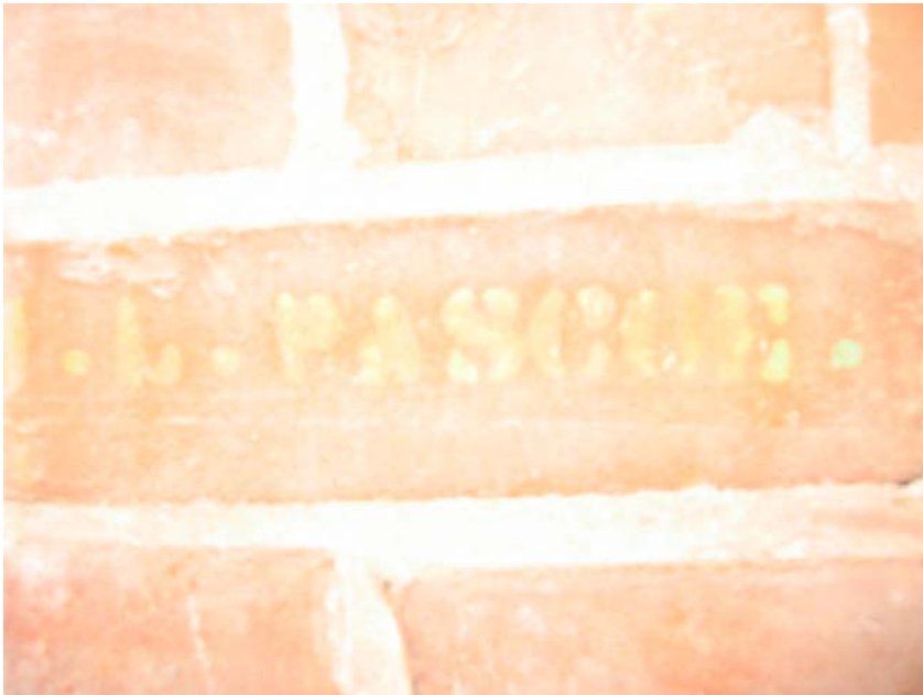
4. Pascoe House, brick with possible builders mark, H.J. PASCOE written on it.
