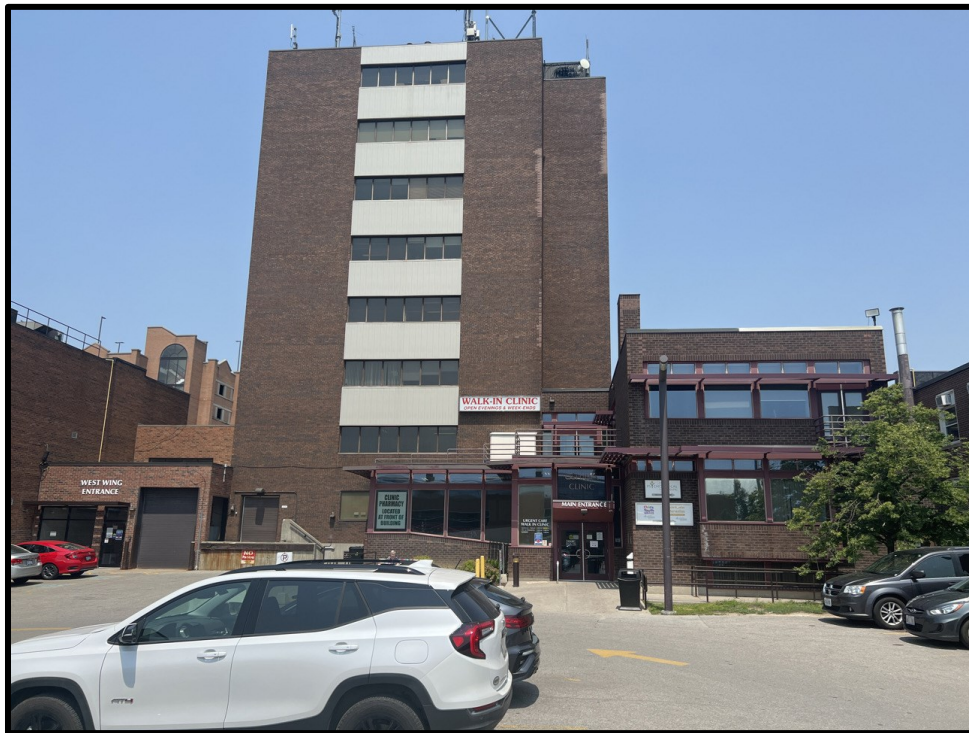
Image 12: View of South Elevation at 117 King Street East (Photo taken on June 19, 2023; Facing North)
