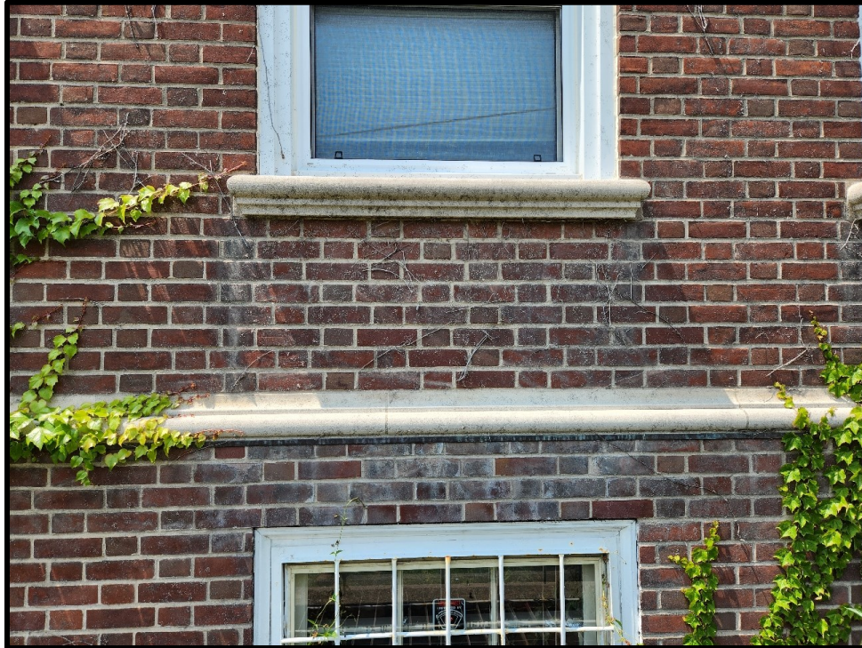
Image 6: Detail of Brick Bond, Torus Moulding and Stone Sill of 1948 East Wing (Photo taken June 19, 2023; Facing Southeast)
