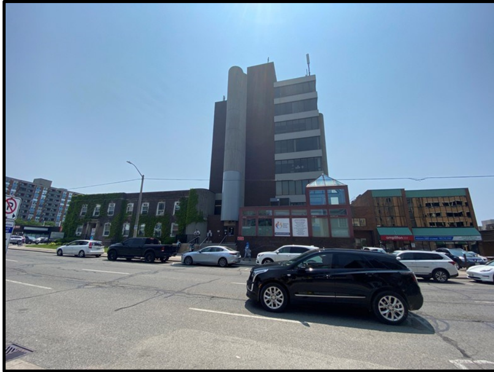
Image 1: Façade of 117 King Street East (Photo taken June 19, 2023; Facing South)
