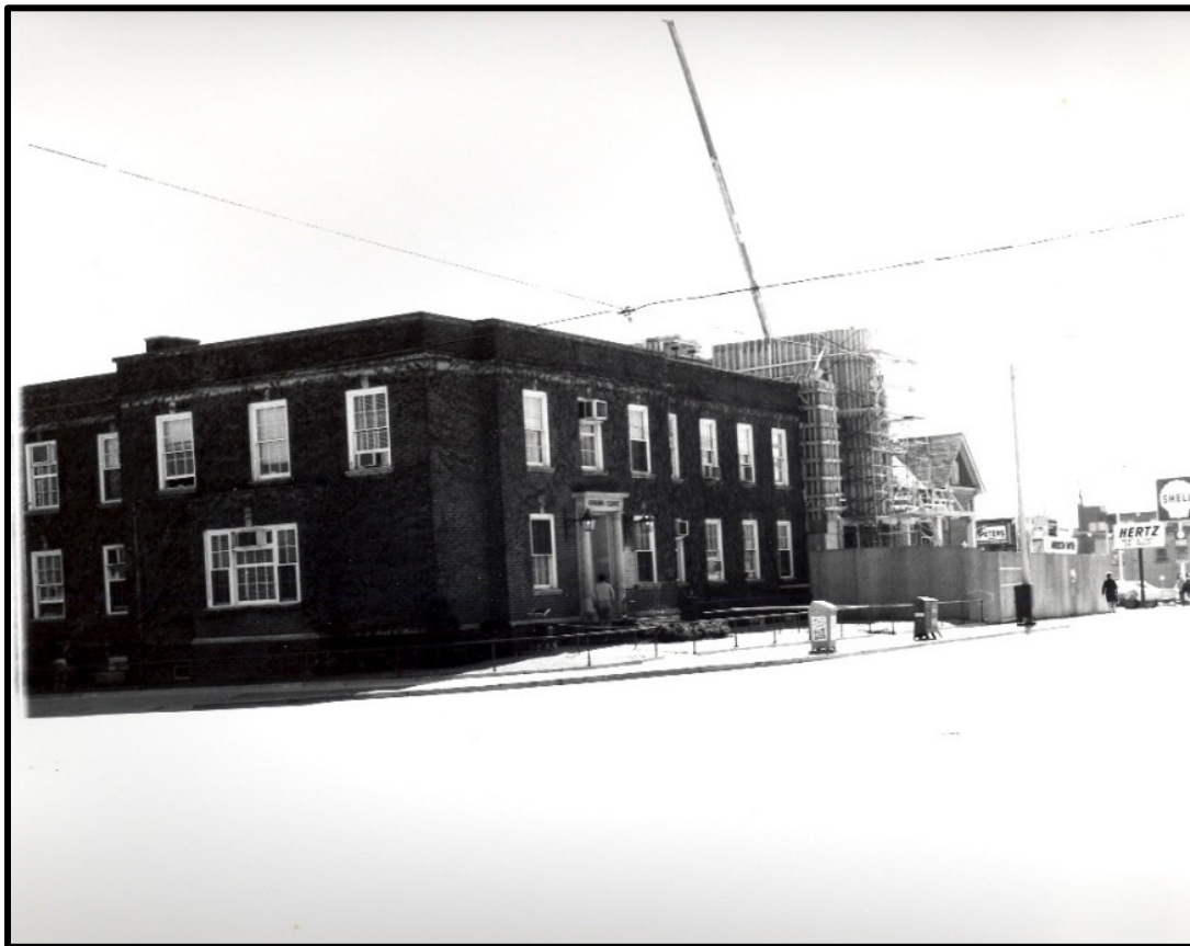
Figure 2: Photograph Showing the Construction of the Tower (Circa 1970) (Thomas Bouckley Collection In Cole 2021:12)
