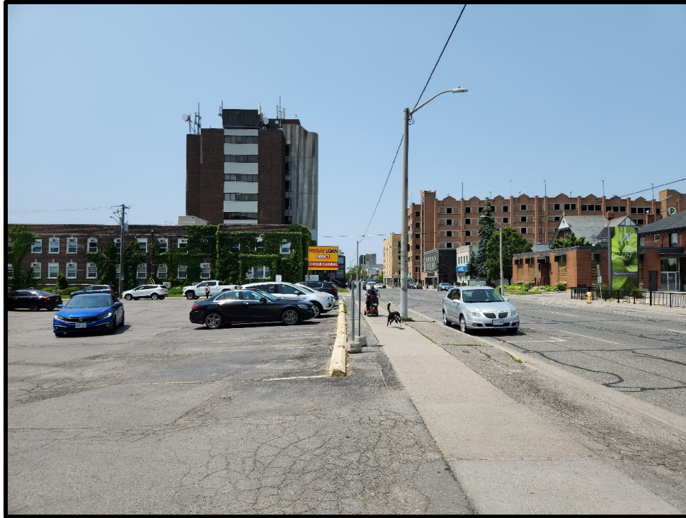
Image 11: View of East Elevation of 117 King Street East (Photo taken on June 19, 2023; Facing West)
