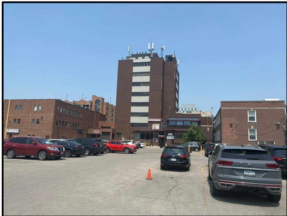
Image 8: South Elevation of 117 King Street East (Photo taken on June 19, 2023; Facing North)
