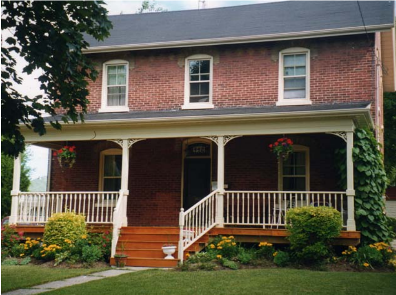
East Façade, 442 King Street East, 1998
