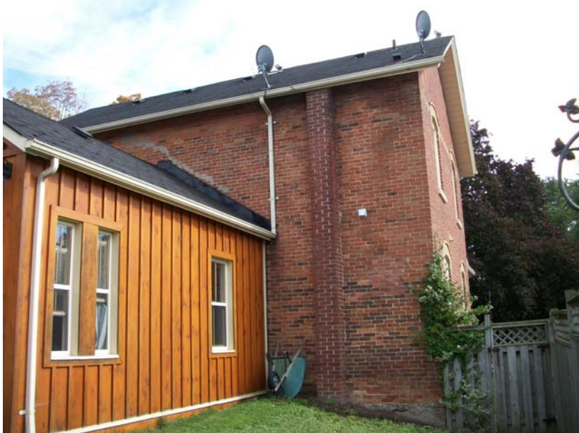
North West Façade, 442 King Street East, September 2010
