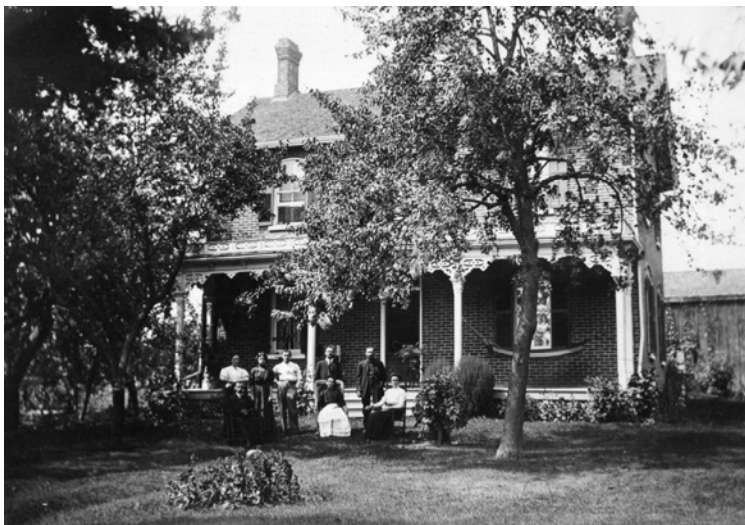
South Façade, 442 King Street East, Oshawa. Circa 1880
