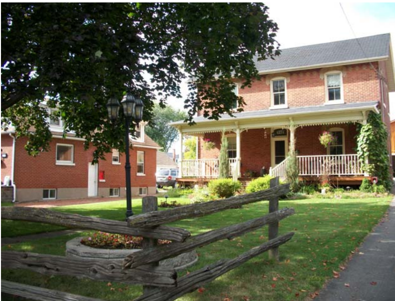
South Façade, 442 King Street East, September 2010
