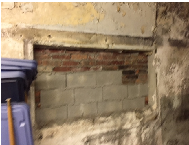
2. Interior wall of the original carriage shed.
