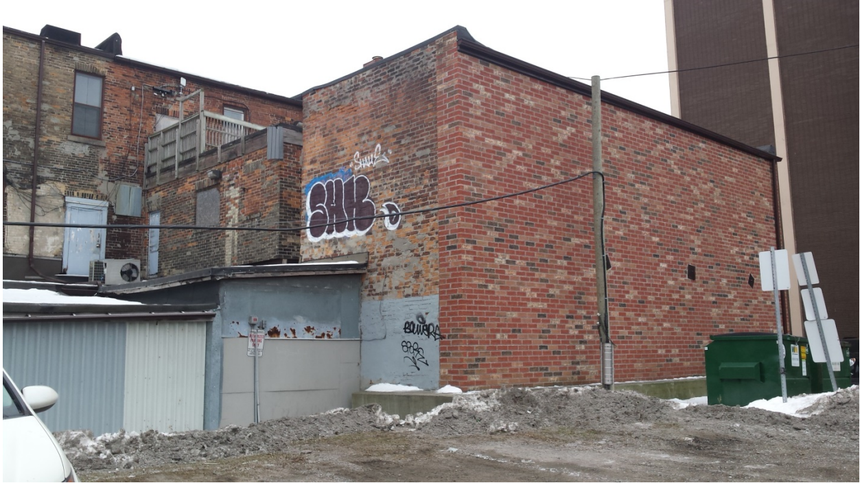
5. Carriage Shed, North East Façade
