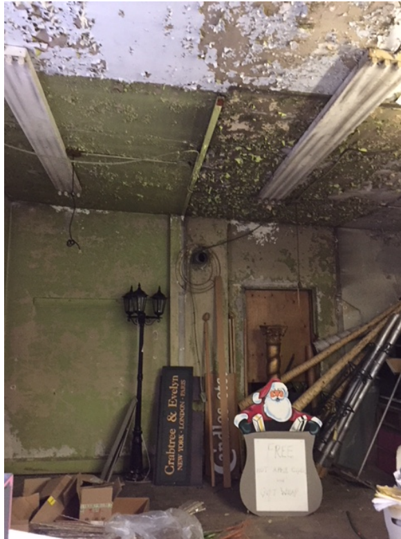
1. Interior, main floor, of the original carriage shed. Currently used for storage for the Gift House when it was in business.
