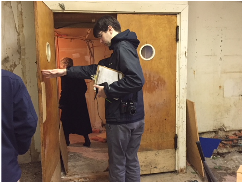
4. Double doors that are located on the second floor of the original carriage shed where it attaches to the main building. These doors lead to a kitchen area that served a café/restaurant that was located here. i.e. Grand Restaurant/Café
