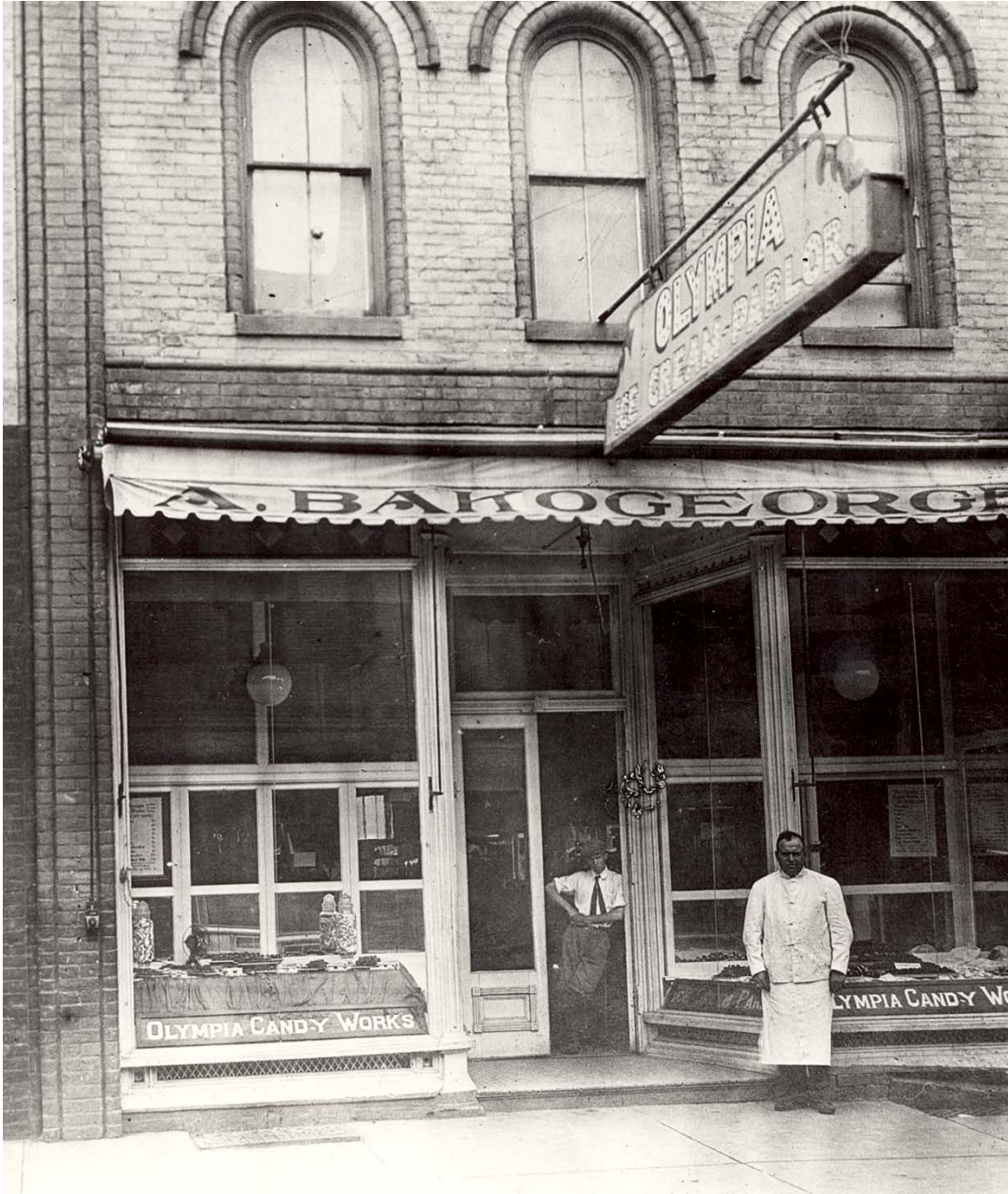
5. 10 King Street East, Olympia Ice Cream Parlour, c. 1910 Note: the dichromatic brick work (buff and red brick)
