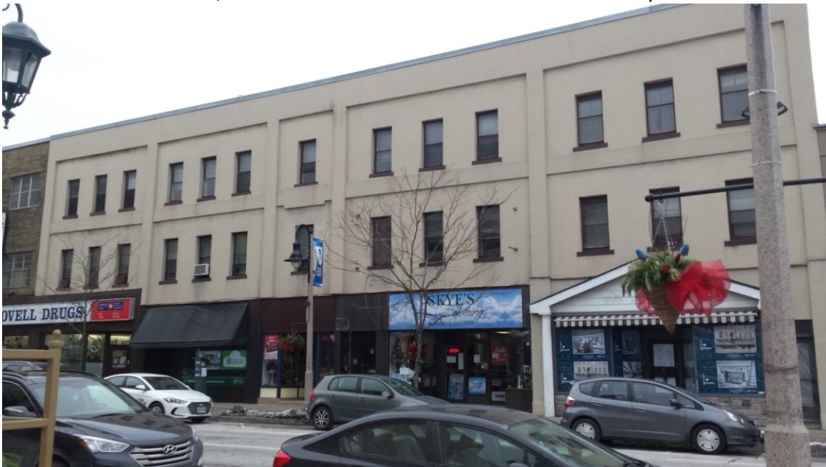
2. Main Façade facing south onto King Street East, looking west
