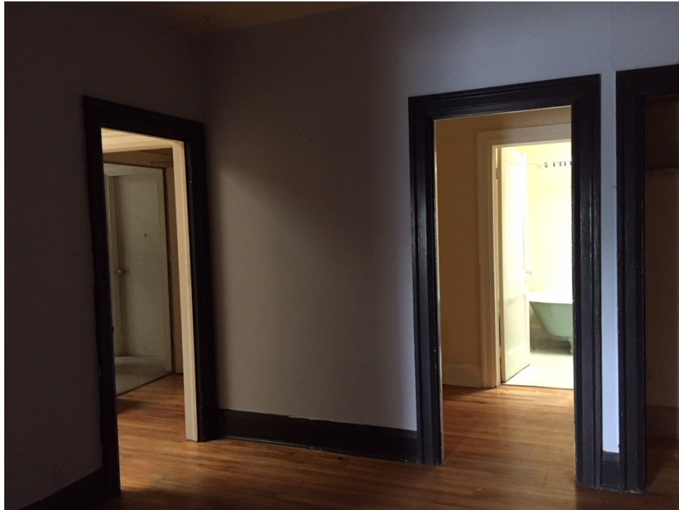
7. Second floor apartment
