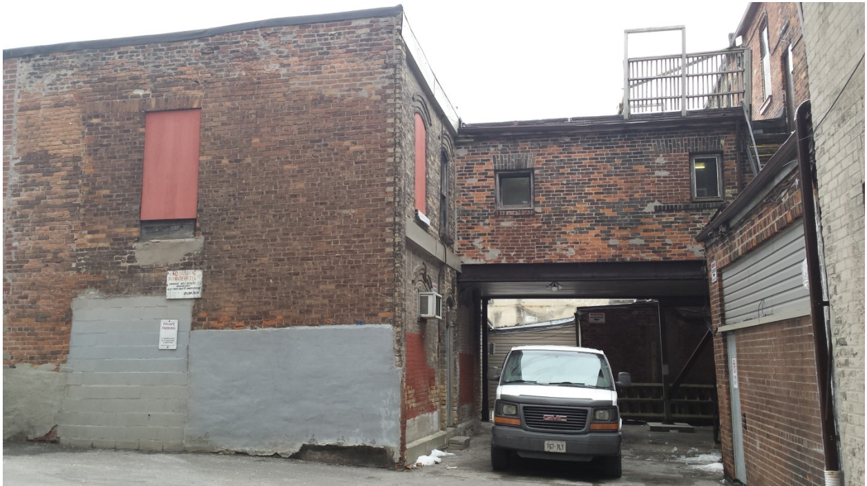
4. Carriage Shed, West Façade, 16 King Street East
