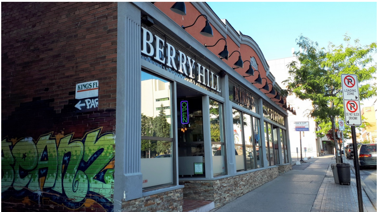
Figure 4 - 78, 80, 82 King Street West, Oshawa. South-West Facade, September 2019
