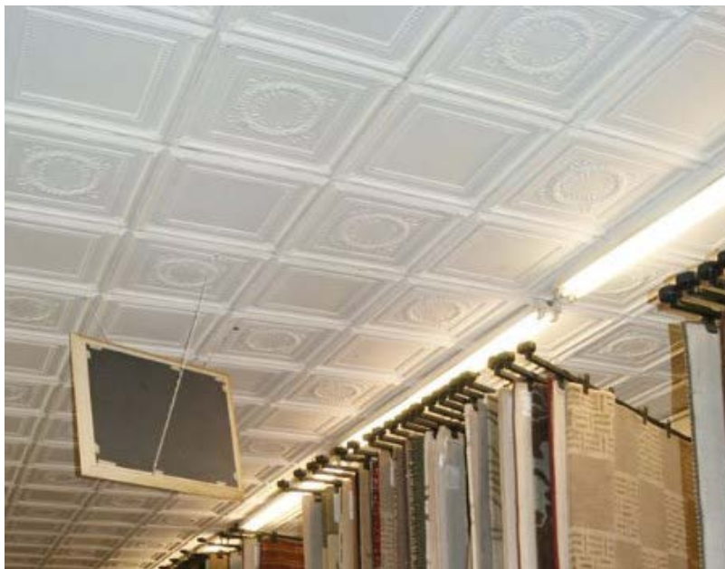
Figure 2 - Tin ceiling tiles made and installed by Pedlar People Ltd., of Oshawa. These ceiling tiles are located in both stores and are original to the building. This represents one of the few examples of these tiles still in place.
