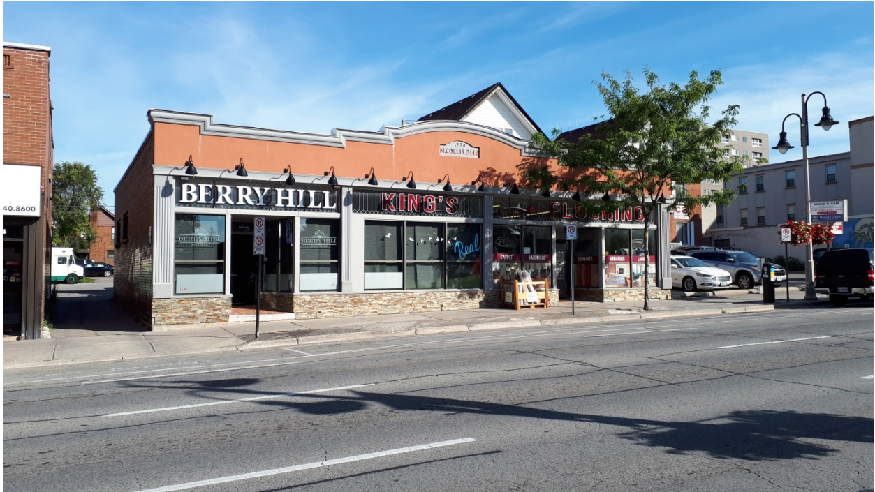
Figure 3 - 78, 80, 82 King Street West, Oshawa. South Facade, September 2019
