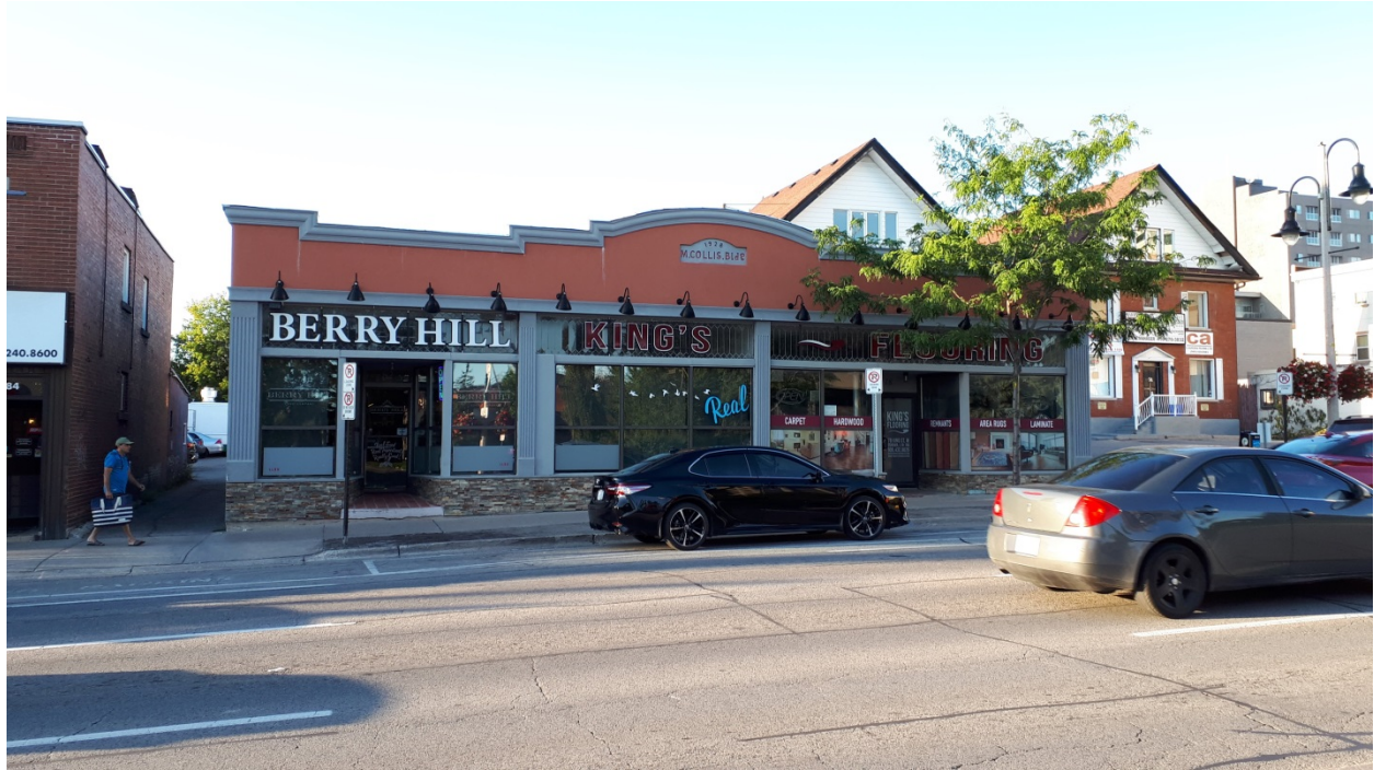
M. Collis Building
