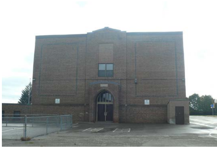
North façade – September 2012
