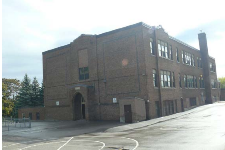
North façade with original BOYS entrance – September 2012
