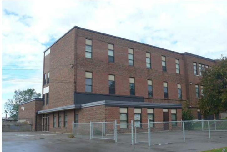
South East Façade – September 2012
