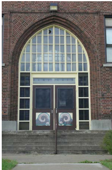
Entranceway East Façade – September 2012
