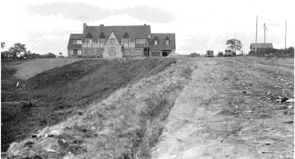
Figure 2: 46 Riverside Drive North, circa 1928/29, during construction. Source: Ted Rundle
