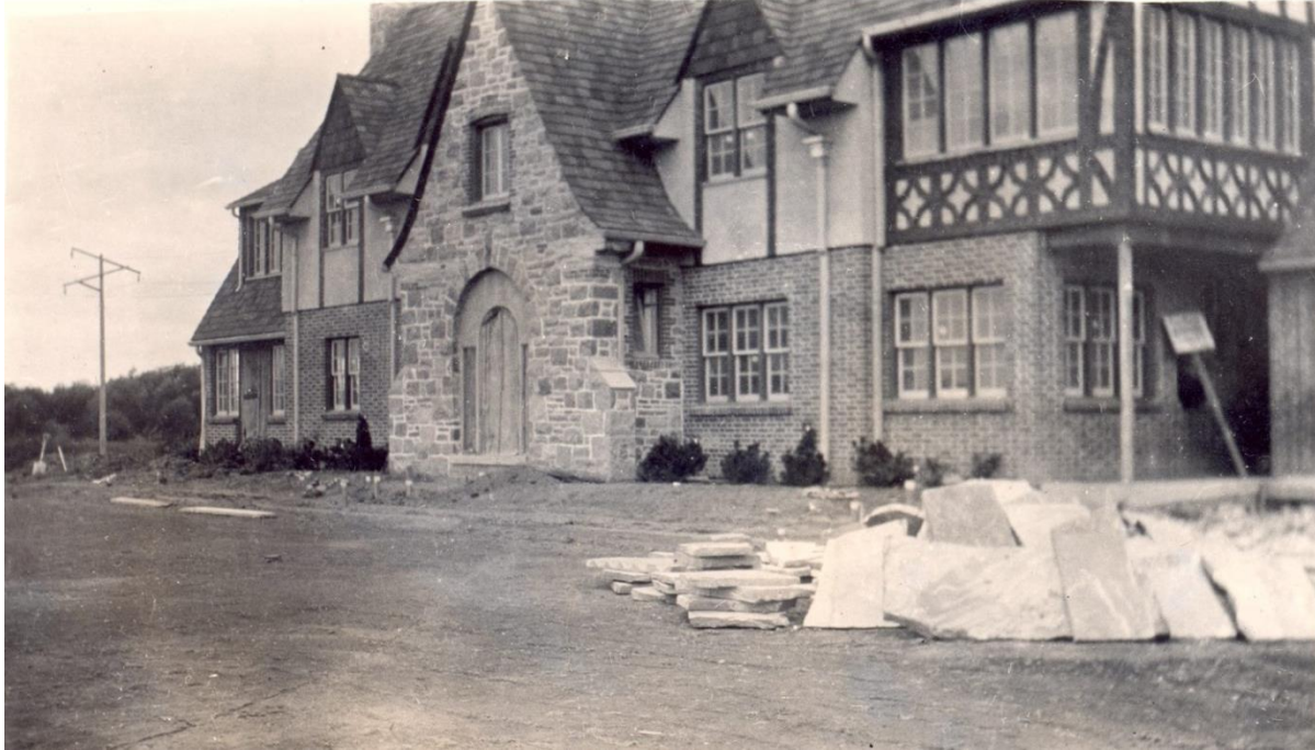
Figure 3: 46 Riverside Drive North, circa 1928/29, during construction. Source: Ted Rundle
