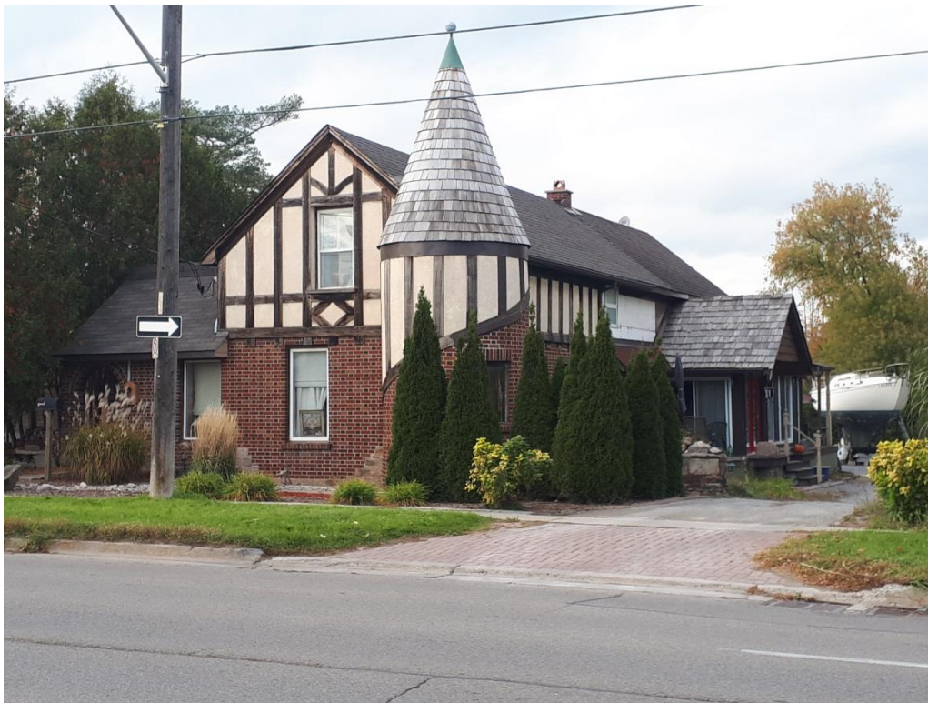
Figure 2: 708 King Street East, The original Gardener's/GateKeeper's House
