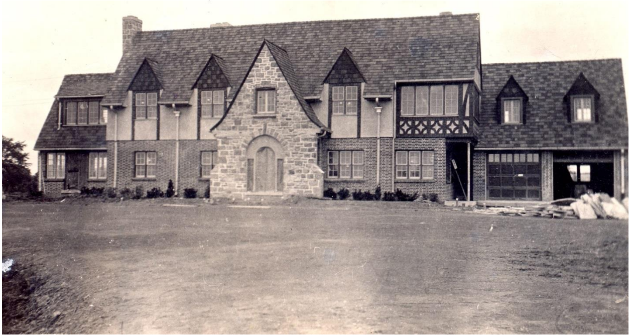
Figure 1: 46 Riverside Drive North, circa 1928/29, during construction. Source: Ted Rundle
