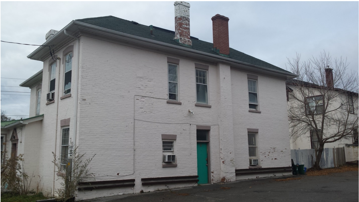
East Façade, Rear of the Building
