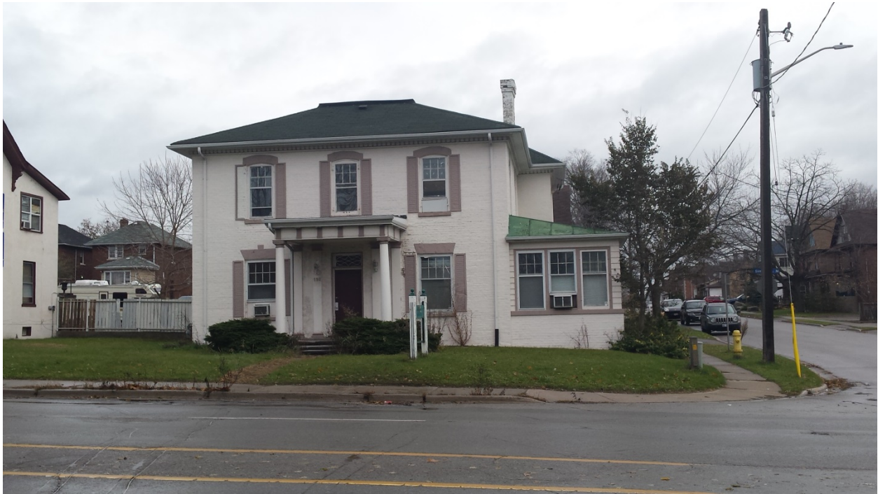
West Façade facing west onto Simcoe Street North
