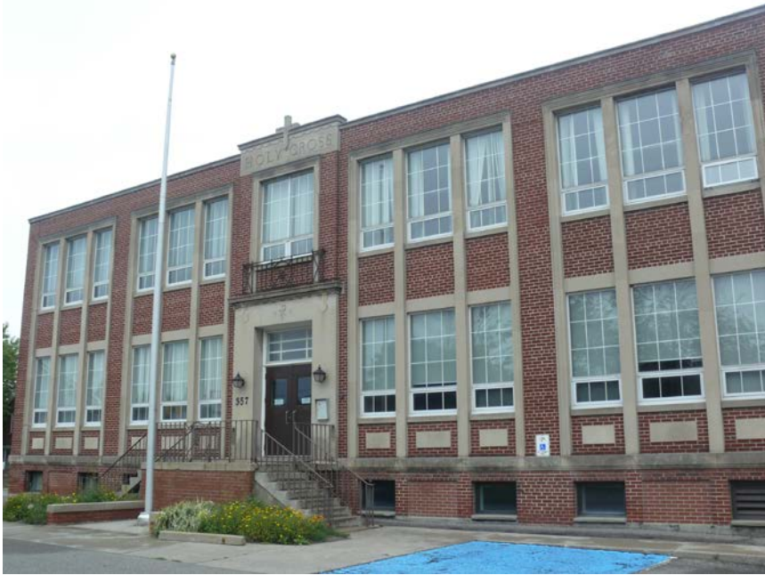
1. West Façade, August 2008
