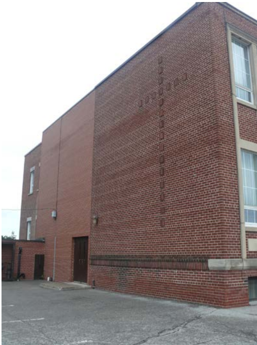
4. North Façade, August 2008
