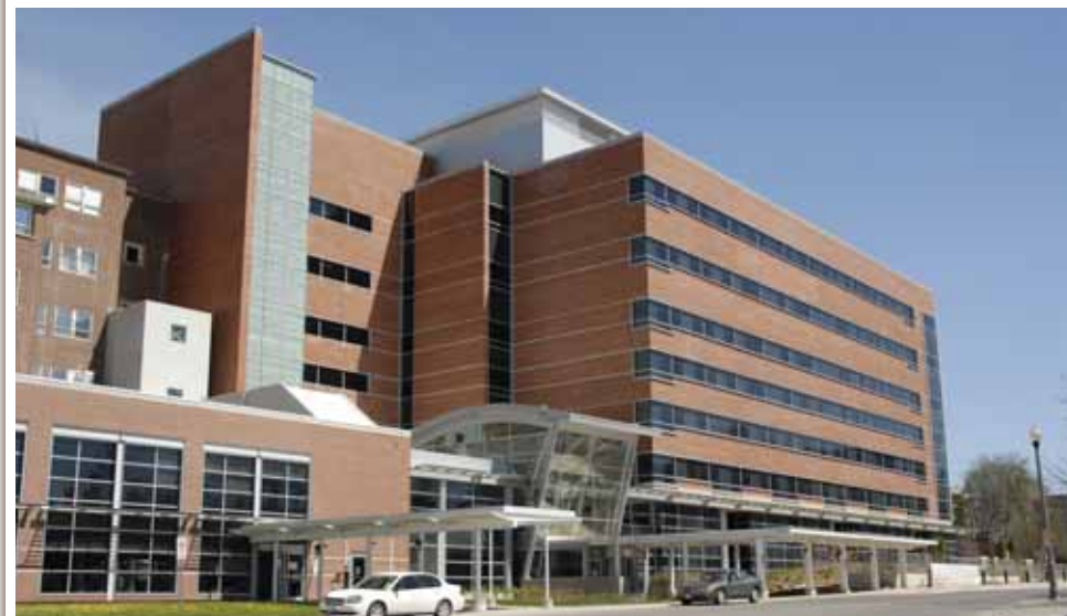
Lakeridge Health Oshawa continues to invest in health care excellence and has recently constructed the Durham Regional Cancer Centre, new dialysis unit and LHEARN centre.
