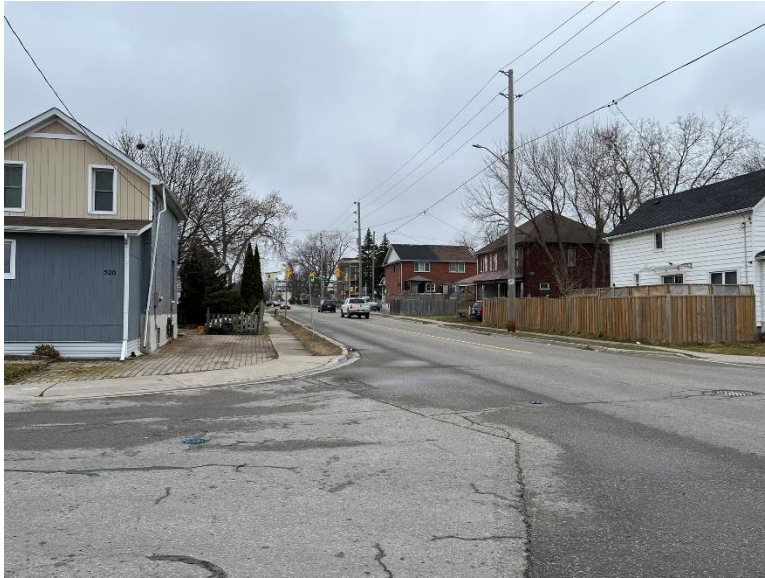
Figure 12: Residential context along First Avenue, looking west from Front Street (A.S.I., 2024)
