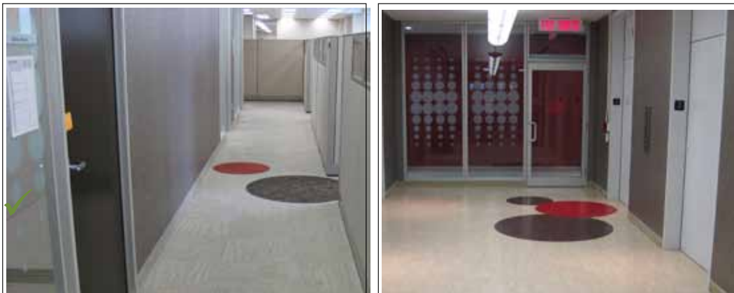
Example of floor surface and elevator door finishes that minimize glare.
