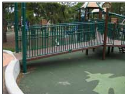
Ramp connected to elevated play components.
