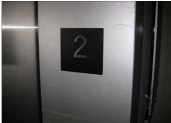
Tactile elevator car identification sign.
