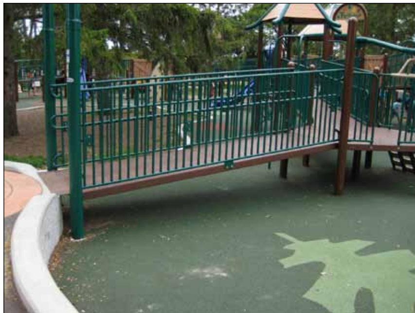
An example of accessible entry / exit point and accessible route leading to elevated play components.
