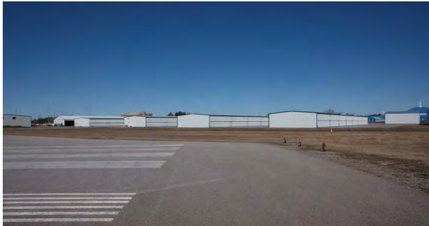
Figure 29: General Aviation Hangar Complex
