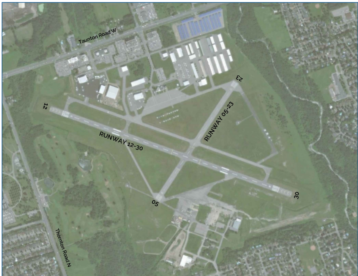
Figure 2.1 - Oshawa Executive Airport Overview
