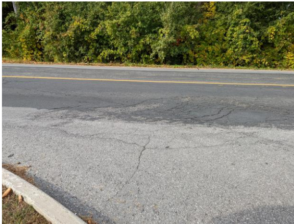
Figure 3: Cracks in Pavement on NB Lane, approx. 90m north of Taunton
