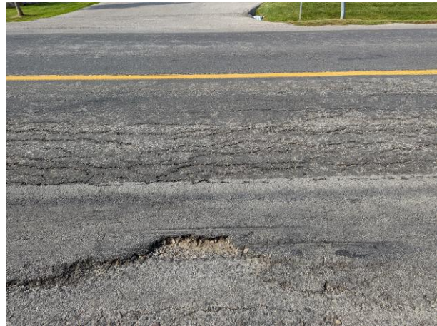
Figure 4: Cracks and Hole in Pavement on NB Lane, approx. 1.1 km south of Conlin
