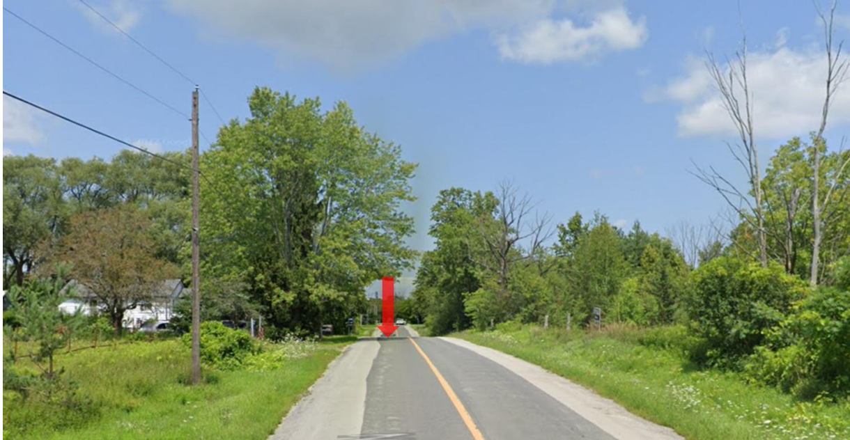
Figure 7: Crest Vertical Curve on Stevenson Rd, Looking North approx. 500m South of Conlin Road
