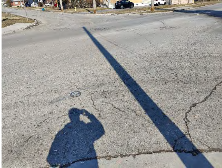
Photograph 19 – First Avenue, in the vicinity of the intersection of Howard Street and First Avenue, looking North, showing moderate to severe random cracking, slight pavement edge cracking, and moderate to severe pavement raveling. Noting severe alligator cracking around manholes and section of patching.
