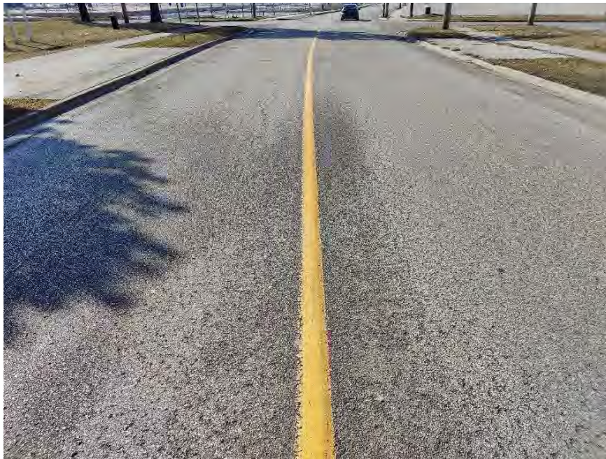
Photograph 20 – First Avenue, approximately 40 m East Howard Street, looking Southwest, showing slight longitudinal and transverse cracking, slight random cracking, slight pavement edge cracking, and slight to moderate pavement raveling.
