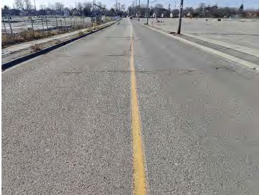
Photograph 17 – First Avenue, approximately 35 m West of Howard Street, looking West, showing moderate to severe longitudinal and transverse cracking associated with moderate random cracking, slight alligator cracking, slight pavement edge cracking, and moderate pavement raveling. Noting moderate random cracking around manholes.
