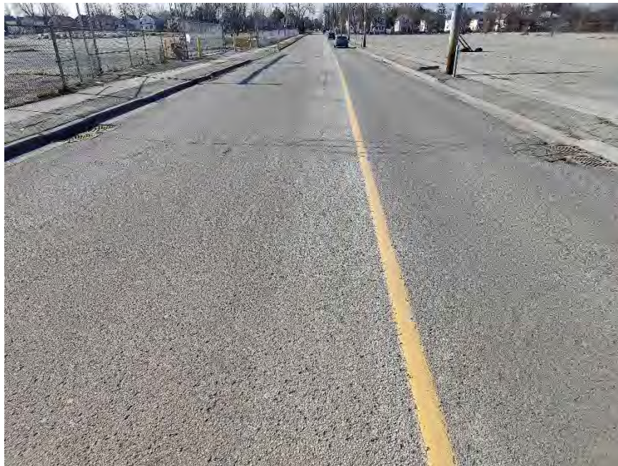
Photograph 16 – First Avenue, approximately 130 m East of Front Street, looking West, showing slight to moderate longitudinal and transverse cracking associated with moderate random cracking, slight to moderate alligator cracking, slight to moderate pavement edge cracking, and moderate to severe pavement raveling. Noting severe alligator cracking and slight random cracking around catch basins.
