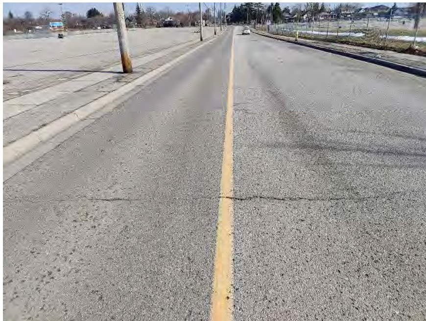
Photograph 12 – First Avenue, approximately 45 m East of Front Street, looking East, showing slight to moderate longitudinal and transverse cracking associated with slight random cracking, slight pavement edge cracking, slight pavement rutting, and moderate pavement raveling.
