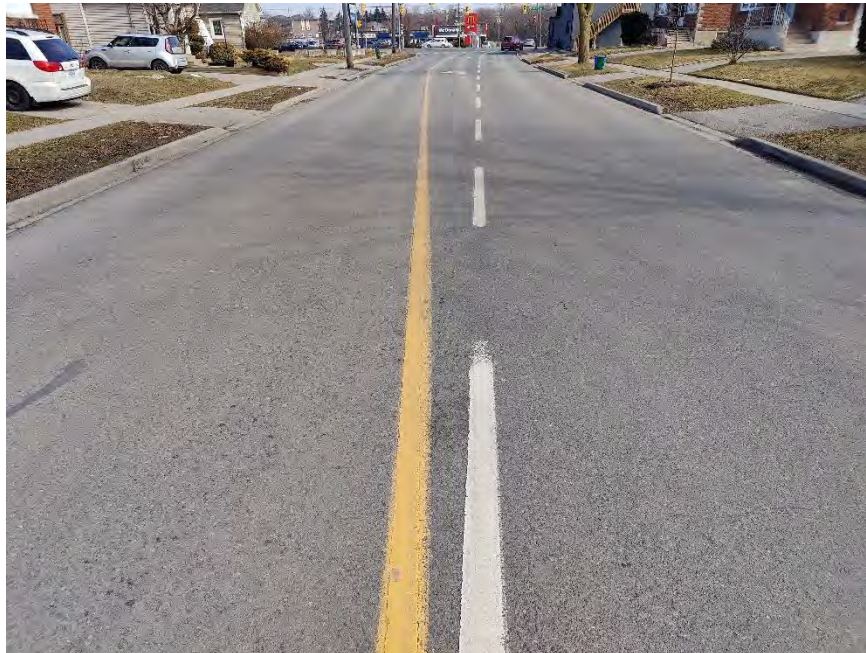
Photograph 28 – McNaughton Avenue, approximately 100 m West of Ritson Road South, looking East, showing slight to moderate longitudinal cracking, slight random cracking, and slight pavement raveling.
