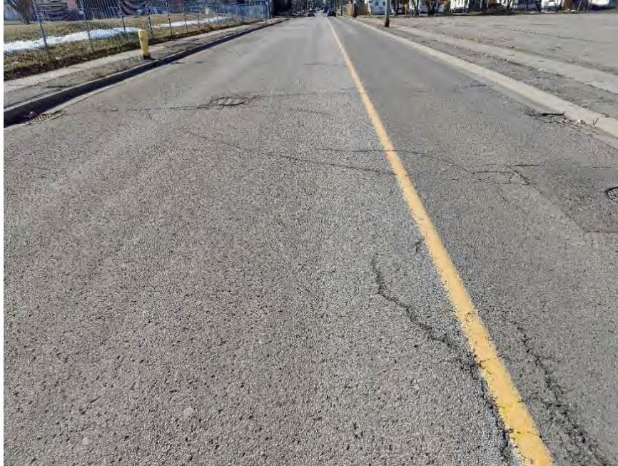
Photograph 13 – First Avenue, approximately 100 m East of Front Street, looking West, showing slight to moderate longitudinal and transverse cracking associated with slight random cracking, slight alligator cracking, slight pavement edge cracking, and moderate to severe pavement raveling. Noting moderate alligator cracking around manhole and catch basin, and utility patching.
