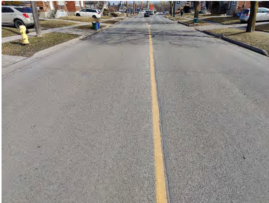
Photograph 26 – McNaughton Avenue, approximately 100 m East of Drew Street, looking East, showing slight longitudinal cracking associated with slight random cracking, and moderate pavement raveling. Noting moderate random cracking around manhole.
