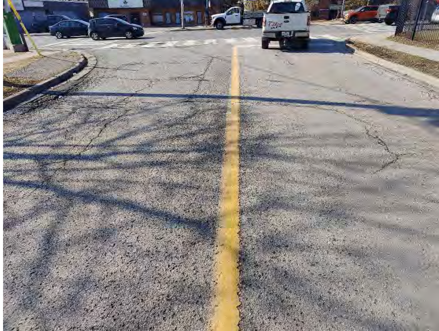
Photograph 1 – First Avenue, approximately 30 m East of Simcoe Street South, looking West, showing moderate to severe longitudinal and transverse cracking associated with slight to moderate random cracking, moderate to severe alligator cracking, moderate to severe pavement edge cracking, and moderate to severe pavement raveling.
