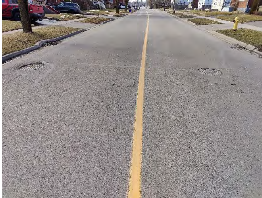
Photograph 27 – McNaughton Avenue, approximately 100 m West of Ritson Road South, looking West, showing slight longitudinal and transverse cracking, slight pavement edge cracking, and slight pavement raveling. Noting slight depression and random cracking around manholes and catch basins, and section of patching.
