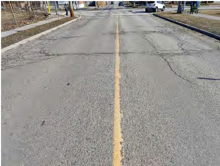
Photograph 6 – First Avenue, approximately 30 m West of Albert Street, looking East, showing moderate longitudinal and transverse cracking associated with moderate to severe alligator cracking, moderate random cracking, slight pavement depressions, severe pavement edge cracking, and moderate to severe pavement raveling.
