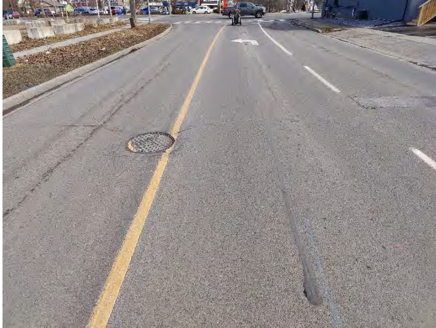
Photograph 29 – McNaughton Avenue, approximately 55 m West of Ritson Road South, looking East, showing slight to moderate longitudinal and transverse cracking associated with slight random cracking, slight pavement edge cracking, and moderate pavement raveling. Noting moderate random cracking around manhole and section of patching.
