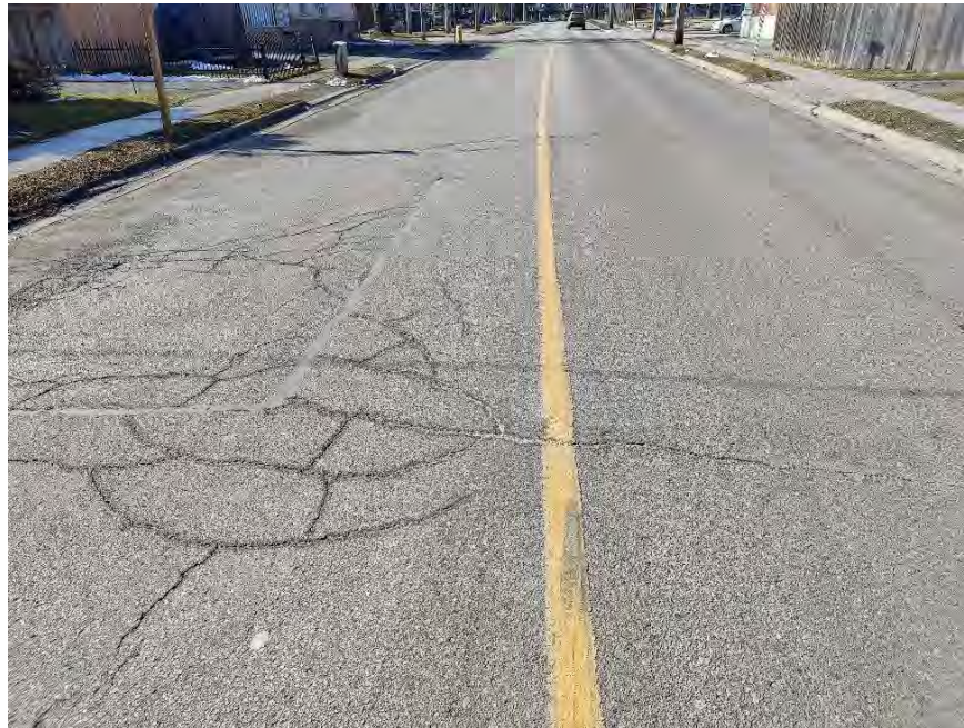
Photograph 8 – First Avenue, approximately 30 m West of Front Street, looking West, showing moderate longitudinal and transverse cracking associated with moderate alligator cracking, slight to moderate random cracking, slight pavement depression, slight to moderate block cracking, slight to moderate pavement edge cracking, and slight pavement raveling. Noting utility patching.
