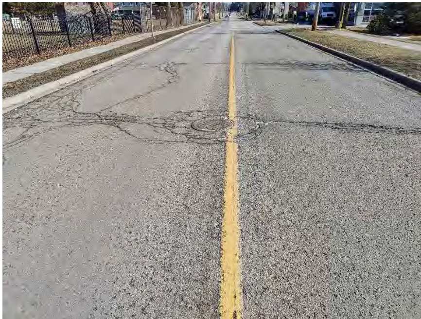
Photograph 4 – First Avenue, approximately 75 m East of Simcoe Street South, looking East, showing slight to moderate longitudinal and transverse cracking associated with moderate to severe alligator cracking, slight to moderate random cracking, severe pavement edge cracking, and moderate to severe pavement raveling. Noting moderate to severe alligator cracking around manhole.
