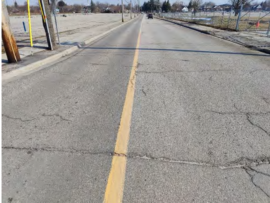
Photograph 11 – First Avenue, in the vicinity of the intersection of Front Street and First Avenue, looking East, showing moderate to severe longitudinal and transverse cracking associated with moderate random cracking, slight pavement edge cracking, and moderate pavement raveling.
