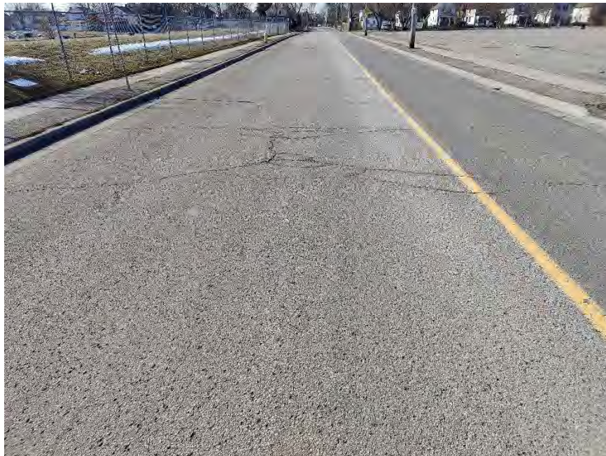
Photograph 14 – First Avenue, approximately 130 m East of Front Street, looking West, showing slight to moderate longitudinal and transverse cracking associated with slight to moderate alligator cracking, slight random cracking, slight pavement edge cracking, and moderate pavement raveling.
