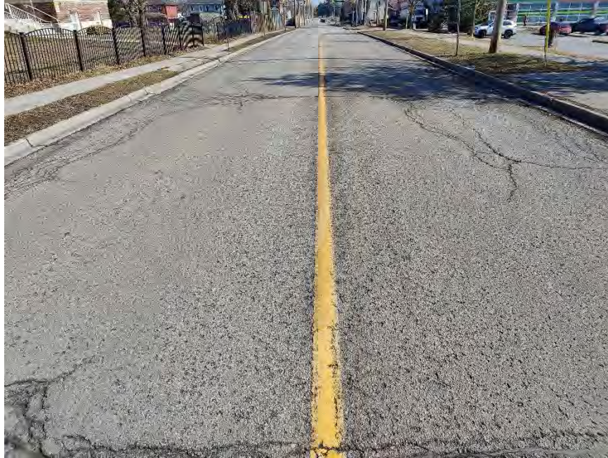
Photograph 3 – First Avenue, approximately 50 m East of Simcoe Street South, looking East, showing slight to moderate longitudinal and transverse cracking associated with moderate to severe alligator cracking, slight to moderate random cracking, severe pavement edge cracking, and moderate to severe pavement raveling.
