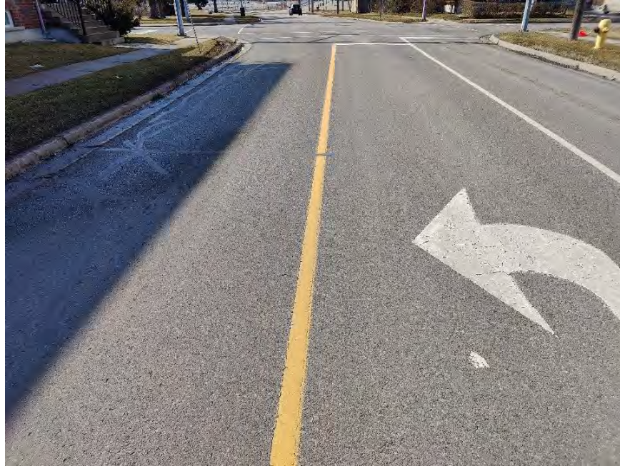
Photograph 23 – McNaughton Avenue, approximately 30 m East of Drew Street, looking West, showing slight to moderate longitudinal and transverse cracking associated with slight random cracking, slight pavement edge cracking, slight to moderate pavement rutting, slight to moderate pavement patching, and slight pavement raveling.
