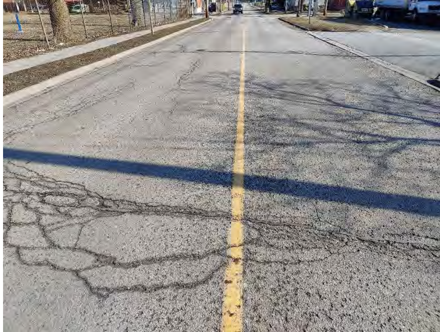
Photograph 5 – First Avenue, approximately 60 m West of Albert Street, looking East, showing moderate to severe longitudinal and transverse cracking associated with severe alligator cracking, slight to moderate random cracking, severe pavement edge cracking, slight pavement depressions, and moderate to severe pavement raveling.
