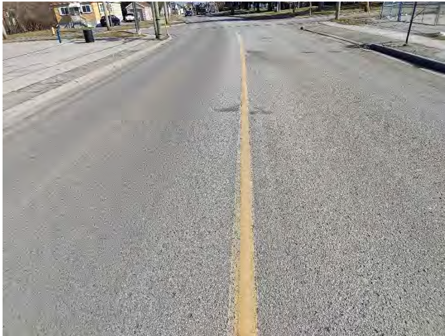
Photograph 18 – First Avenue, approximately 35 m West of Howard Street, looking East, showing slight to moderate transverse cracking, slight pavement edge cracking, and slight to moderate pavement raveling.
