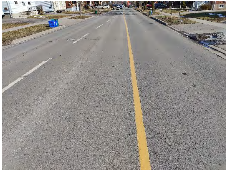
Photograph 24 – McNaughton Avenue, approximately 30 m East of Drew Street, looking East, showing slight to moderate longitudinal and transverse cracking associated with slight random cracking, slight pavement edge cracking, slight pavement rutting, and slight pavement raveling. Noting patching around manhole.
