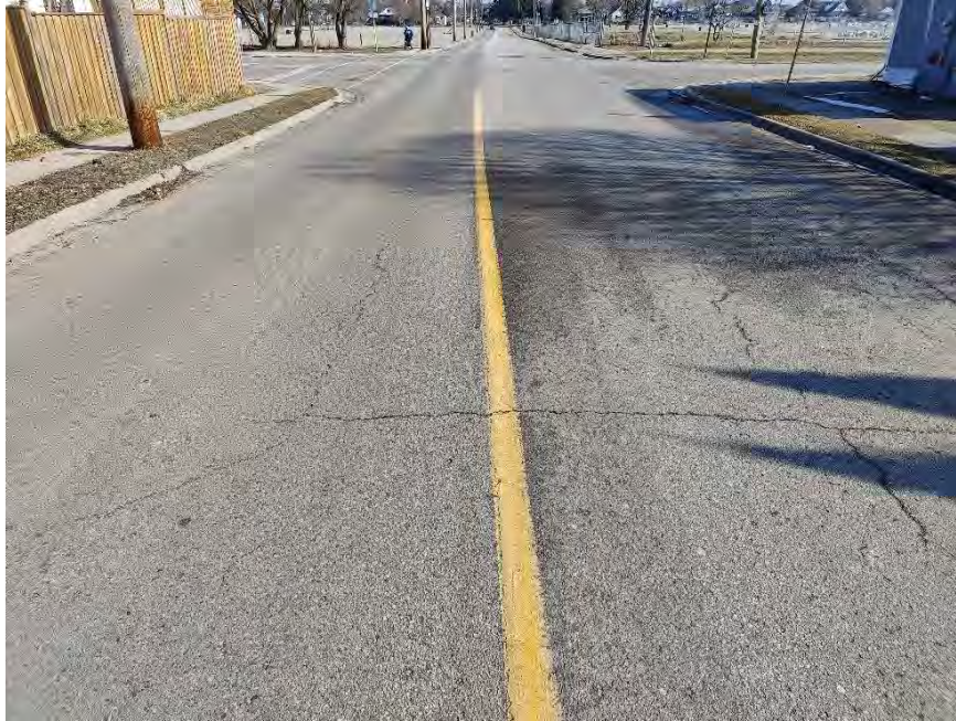
Photograph 9 – First Avenue, approximately 30 m West of Front Street, looking East, showing slight to moderate longitudinal and transverse cracking associated with slight random cracking, slight alligator cracking, slight to moderate pavement edge cracking, slight pavement rutting, and moderate to severe pavement raveling.
