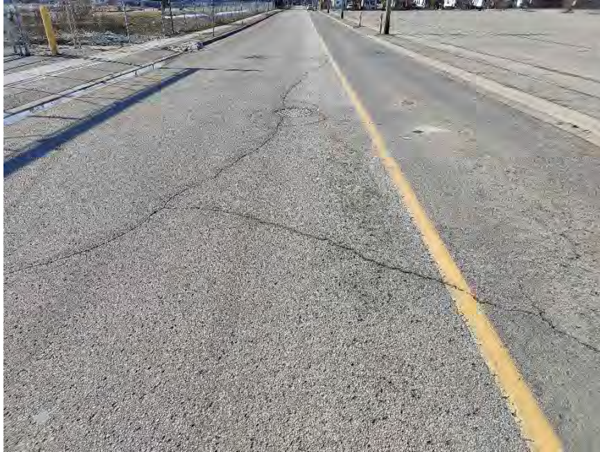
Photograph 15 – First Avenue, approximately 105 m West of Howard Street, looking West, showing moderate longitudinal and transverse cracking associated with moderate random cracking, slight pavement edge cracking, and moderate to severe pavement raveling. Noting moderate random cracking and patching around manholes.
