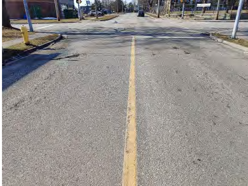
Photograph 7 – First Avenue, approximately 25 m East of Albert Street, looking West, showing moderate longitudinal and transverse cracking associated with moderate random cracking, slight alligator cracking, slight to moderate potholes, slight pavement edge cracking, and moderate pavement raveling. Noting moderate alligator cracking around manholes, slight random cracking around catch basin, and utility patching.
