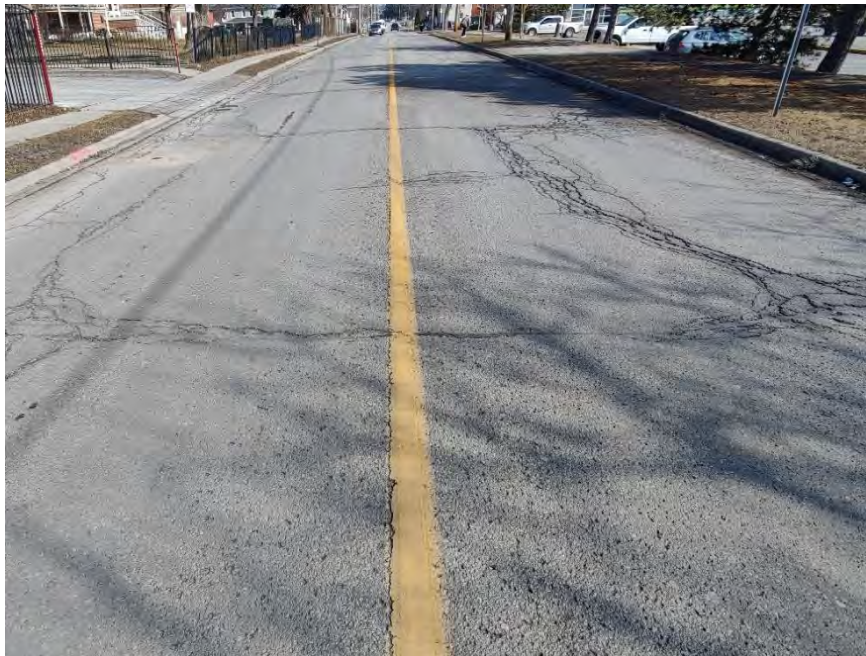
Photograph 2 – First Avenue, approximately 30 m East of Simcoe Street South, looking East, showing moderate to severe longitudinal and transverse cracking associated with moderate to severe alligator cracking, moderate random cracking, severe pavement edge cracking, and moderate to severe pavement raveling.
