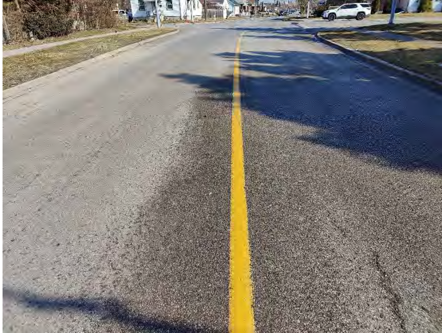
Photograph 21 – First Avenue, approximately 40 m East Howard Street, looking Northeast, showing slight to moderate longitudinal and transverse cracking associated with slight random cracking, slight alligator cracking, slight pavement edge cracking, and moderate pavement raveling.
