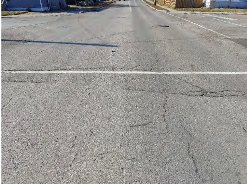
Photograph 10 – First Avenue, in the vicinity of the intersection of Front Street and First Avenue, looking West, showing moderate longitudinal and transverse cracking associated with moderate to severe random cracking, slight alligator cracking, moderate construction joint cracking, and slight to moderate pavement raveling. Noting slight to moderate random cracking around manholes.
