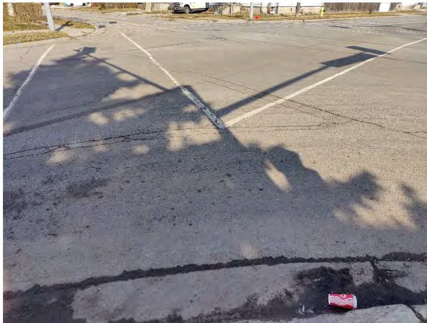
Photograph 22 – First Avenue, in the vicinity of the intersection of Drew Street and First Avenue, looking North, showing slight to moderate longitudinal and transverse cracking associated with moderate random cracking, slight to moderate alligator cracking, slight pavement edge cracking, moderate to severe construction joint cracking, and moderate pavement raveling. Noting severe alligator cracking around manholes and utility patching.
