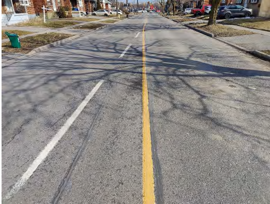
Photograph 25 – McNaughton Avenue, approximately 65 m East of Drew Street, looking East, showing moderate longitudinal cracking associated with slight random cracking, slight pavement edge cracking, slight to moderate pavement rutting, and slight to moderate pavement raveling.
