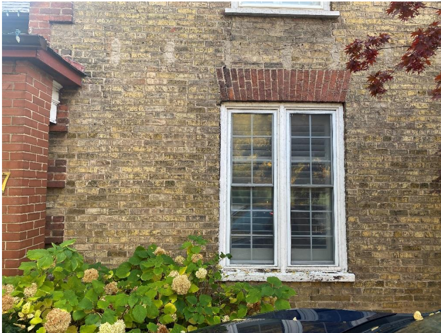
Figure 22: A former casement window on the northern elevation (A.S.I., 2024).
