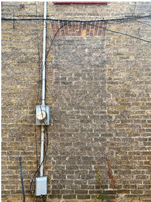
Figure 21: A bricked in window on the western elevation (A.S.I., 2024).
