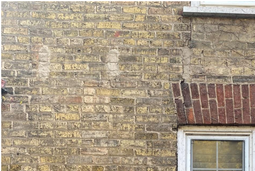
Figure 36: Detail view of the markings on the brick in the northern façade indicating an early covered porch (A.S.I., 2024).
