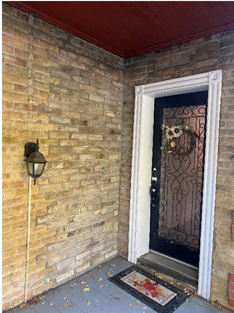
Figure 37: The present-day front door and the location of the original front door to the left. (A.S.I., 2024). Note the different colour brick.
