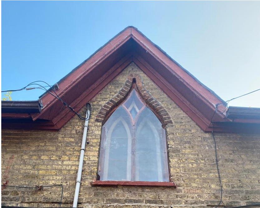
Figure 24: Detail view of the ogee window in the western façade (A.S.I., 2024).
