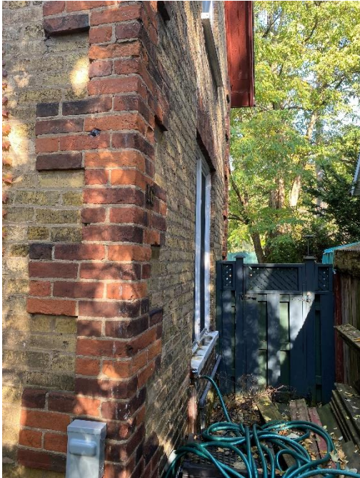
Figure 20: Detail view of the quoining on the eastern elevation showing the dichromatic brick (A.S.I., 2024).
