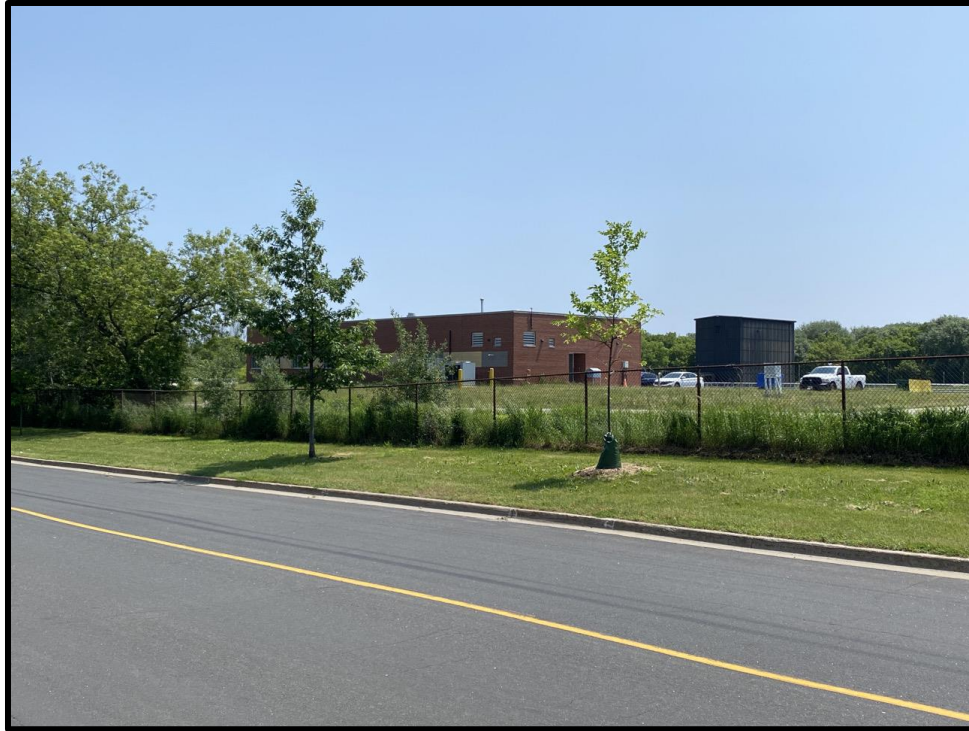
Image 15: Adjacent Wastewater Treatment Plant (Photo taken on June 13, 2023; Facing Southeast)
