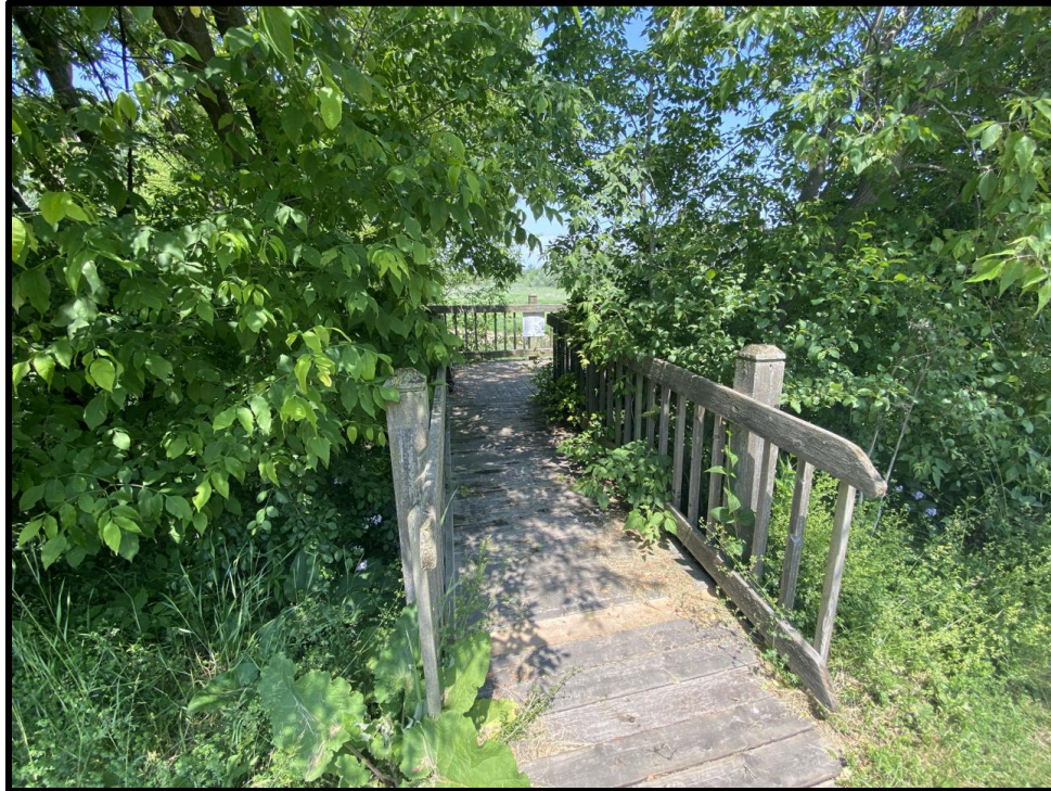
Image 8: Viewing Platform Accessed from Sidewalk (Photo taken on June 13, 2023; Facing North)
