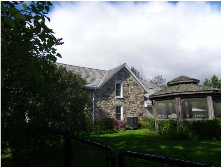
East Façade, 840 Howden Road, Oshawa, September 2010
