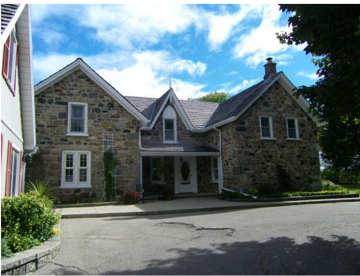
West Façade, North Stone Addition, September 2010
