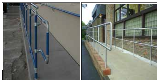
Figure 7b: Handrail Returns to Wall
