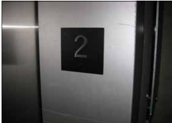
Tactile elevator car identification sign.
