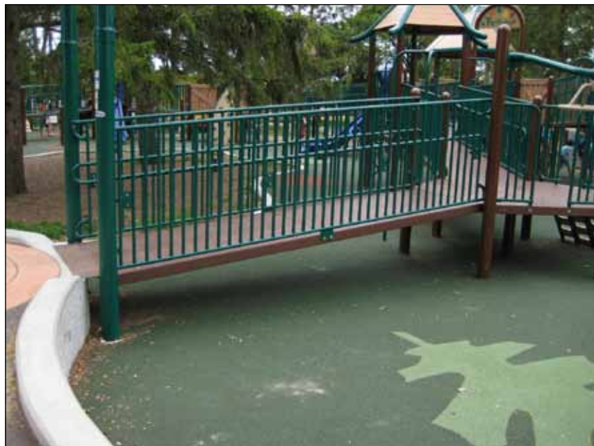
An example of accessible entry / exit point and accessible route leading to elevated play components.
