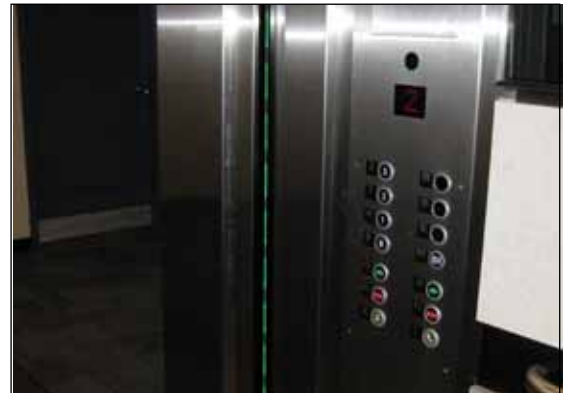
Elevator sensor door and floor registration buttons.
