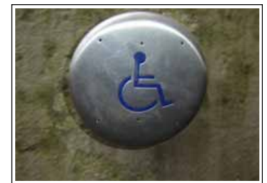
Example of circular power door operator control.
