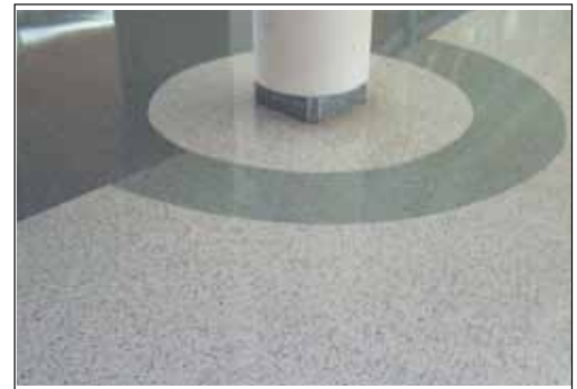
Where a structural column / support may be within an accessible route, a colour contrasted floor surface at base helps identify its location to prevent a potential bumping hazard.
