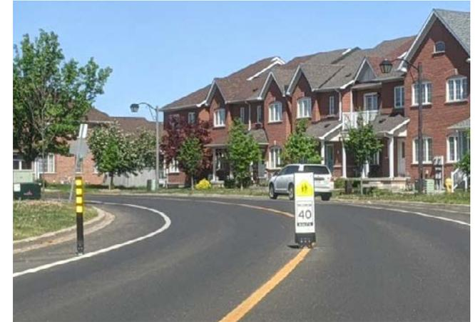
Example of a flexible bollard with delineators
