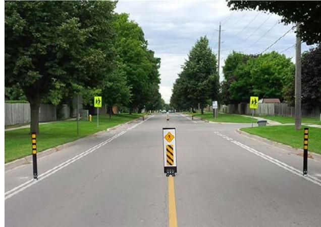
Example of a flexible bollard with delineators
