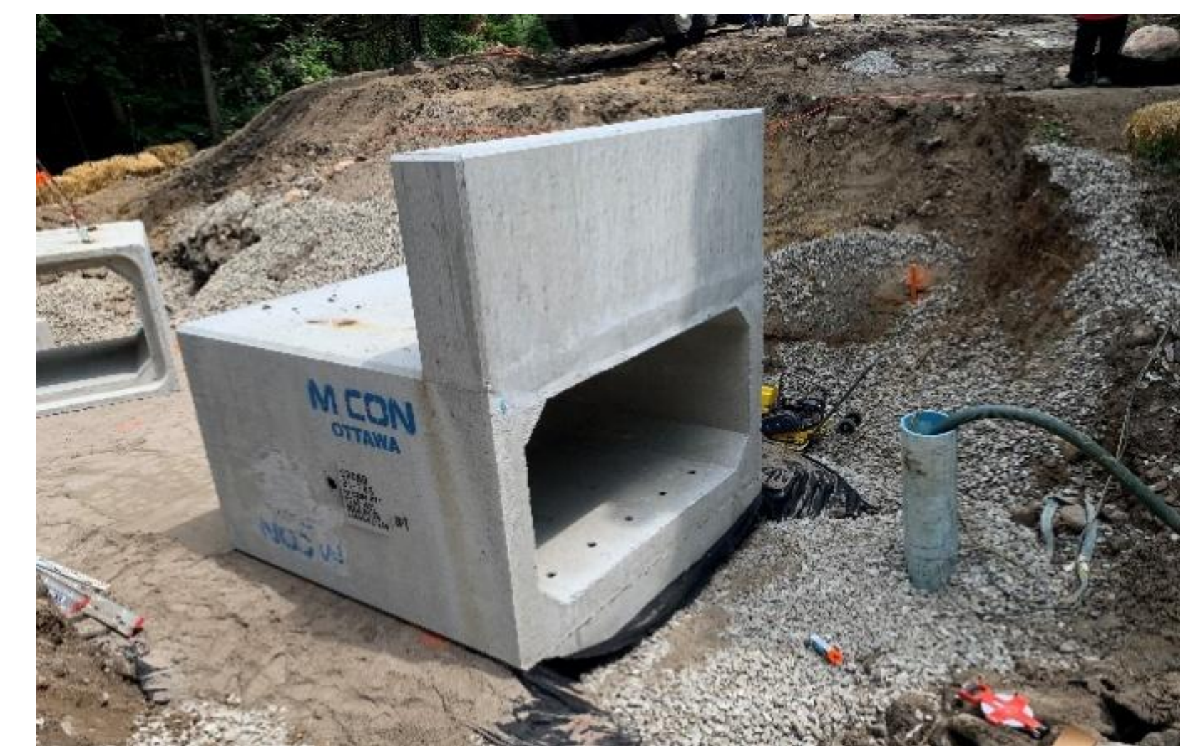
Typical Concrete Box Culvert Construction
