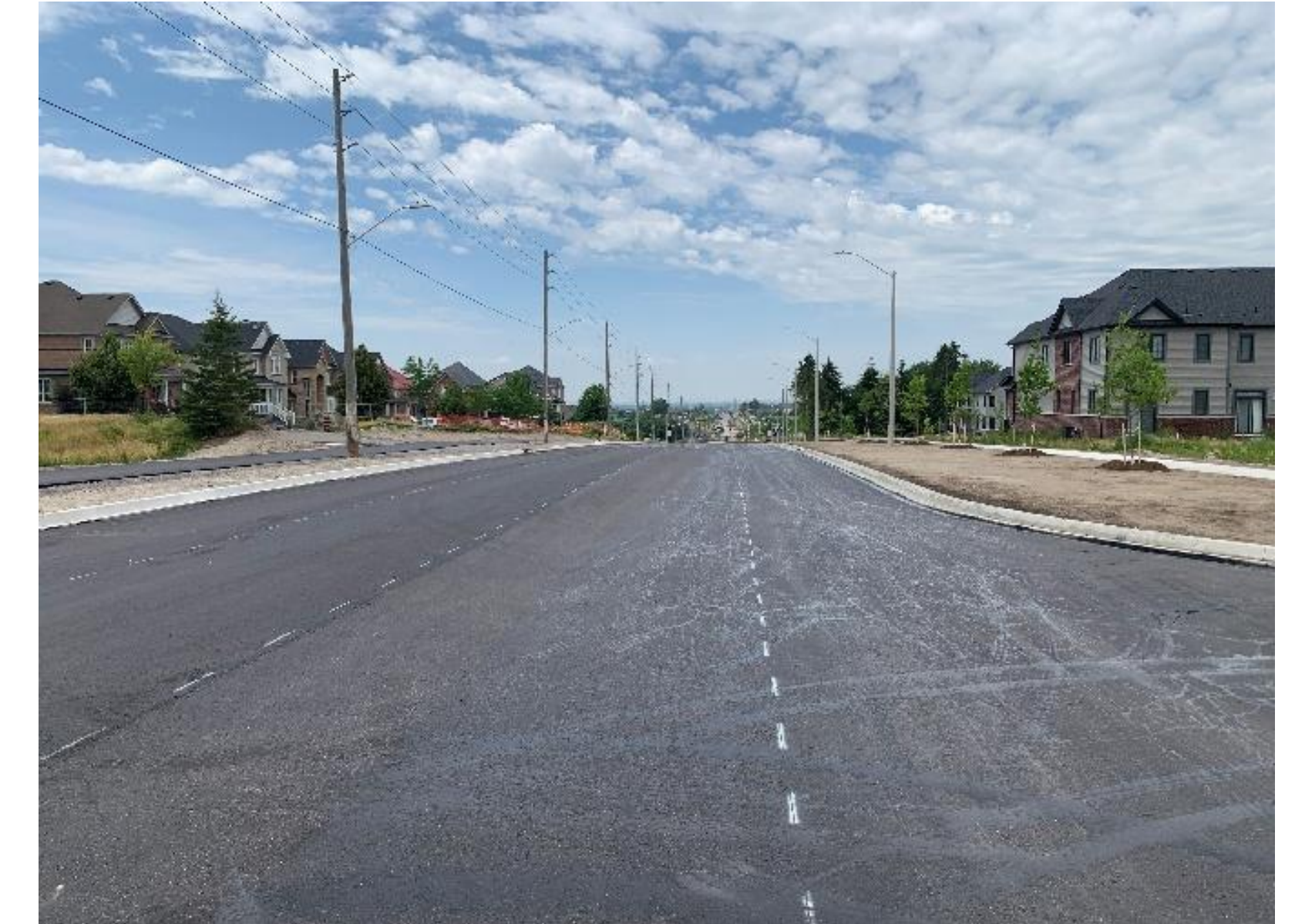
4-Lane Widening of Conlin Road E. Under construction east of Grandview
