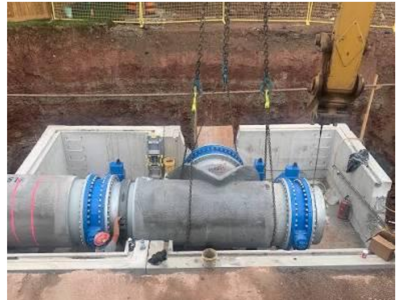
Typical Water Feedermain and Valve Chamber
