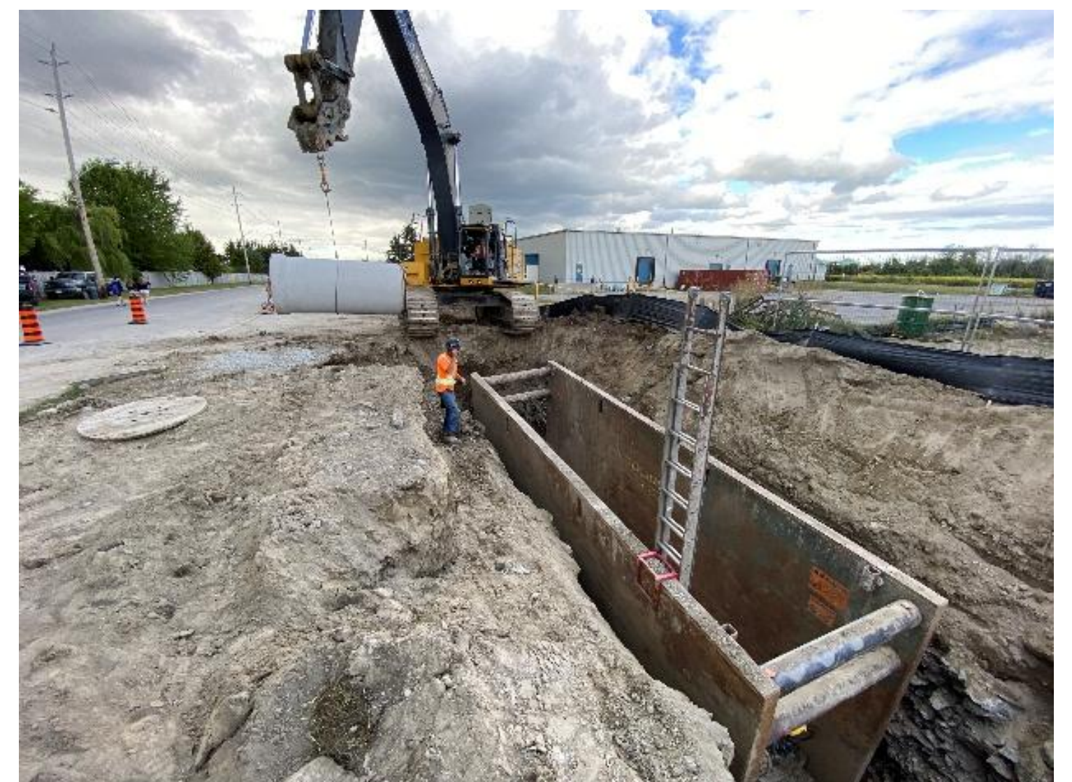
Typical Deep Sanitary Sewer Installation
