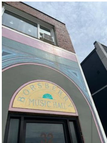
Figure Fourteen: "Borsberry Music Hall" (Brian Romagnoli, 31 Celina St.) – Water damage and discoloration from air conditioning
