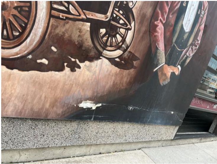
Figure Seven: "General Motors of Canada" (John Hood, Go Bus Station, 47 Bond St.) – Impact damage, cracks, steaks, and peeling
