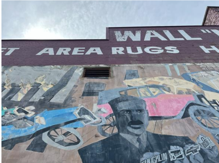
Figure Twenty-three: "Driving Force" (Rudolf Stussi, 22 Athol St. East) – Cracks, chips and streaks
